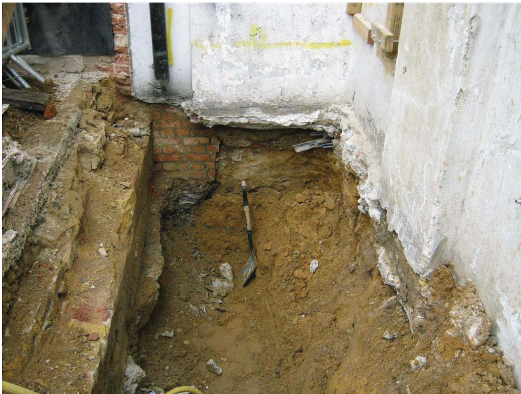
Underpinning Pit 2 Looking East
