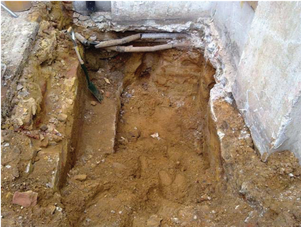
Underpinning Pit 1 Looking North
