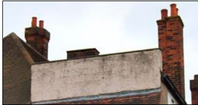
Plate 17: multi-flue chimneys
