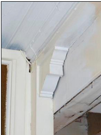
Plate 14: Semi-ornate brackets in the landing.
