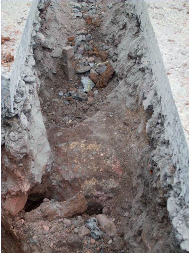
Plate 3: Mortar bonded sandstone blocks with iron bar in background
