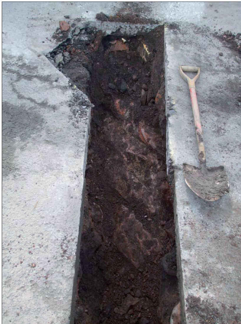
Plate 2: Mortar bonded sandstone blocks in Trench 3
