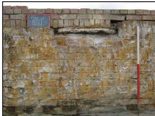
Plate O. View of Opening [612] Looking West
