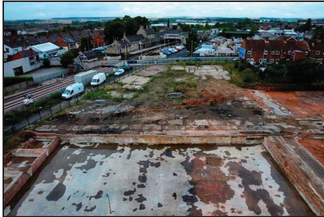
Plate R. View Railway Tracks (695) and (696) Looking West
