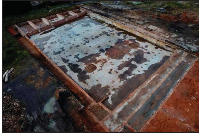
Plate N. View of Room 13 Looking Southwest
