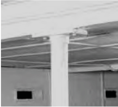
Figure 5. Column prop and securing plate in situ (after Patrick 2004)
