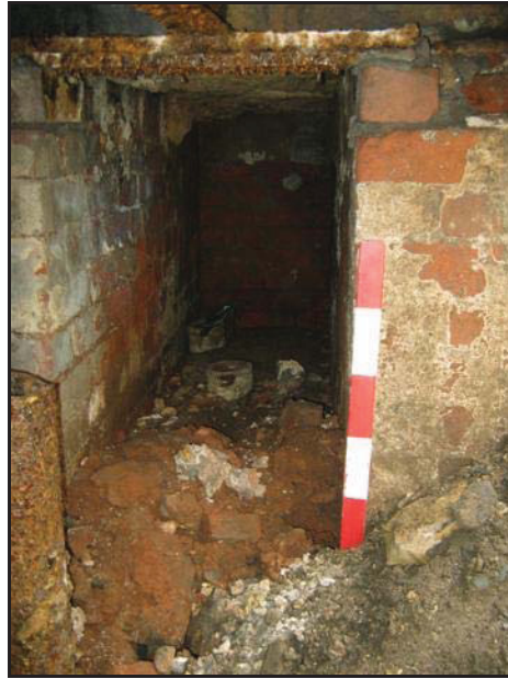
Plate G. View of Tunnel within Chamber
