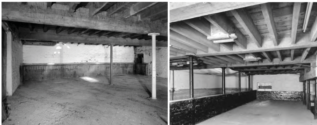
Figure 2 Two examples of cast iron column props used in malting. 2b shows varied heights to be expected.
