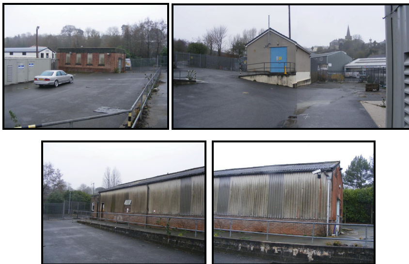
PLATE O: View of the WPD depot in the detached portion of the proposed development site
