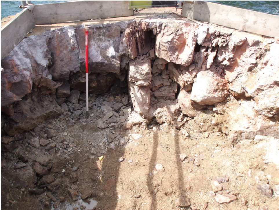
PLATE 3 Concrete layer over sandstone surface over fractured rubble fill with rough blocks, to right of photograph, indicating the original harbour wall construction
