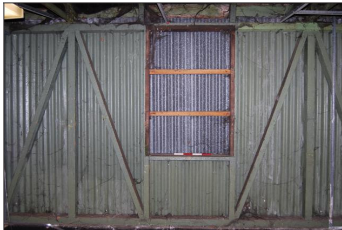
Plate 8: Hut 2 Blocked Window and Wooden Frame
