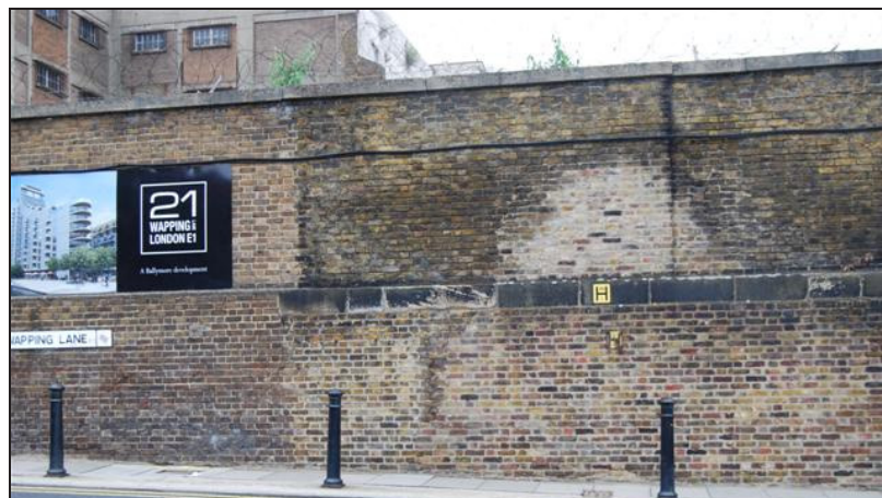
Plate 13: Perimeter Wall Along Wapping Lane, Showing Change of Build
