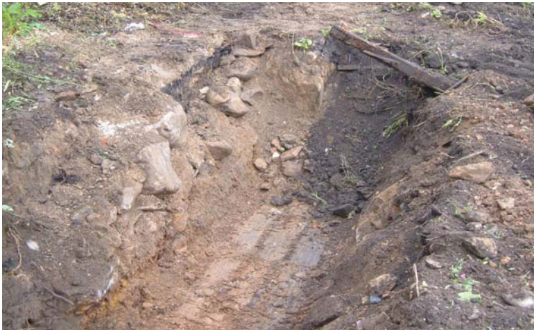
Plate 1: Foundation Trench 2 showing demolition in-fill and made-ground
