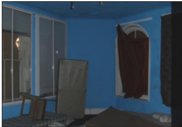
Plate 11: Room F2 Looking Southeast
