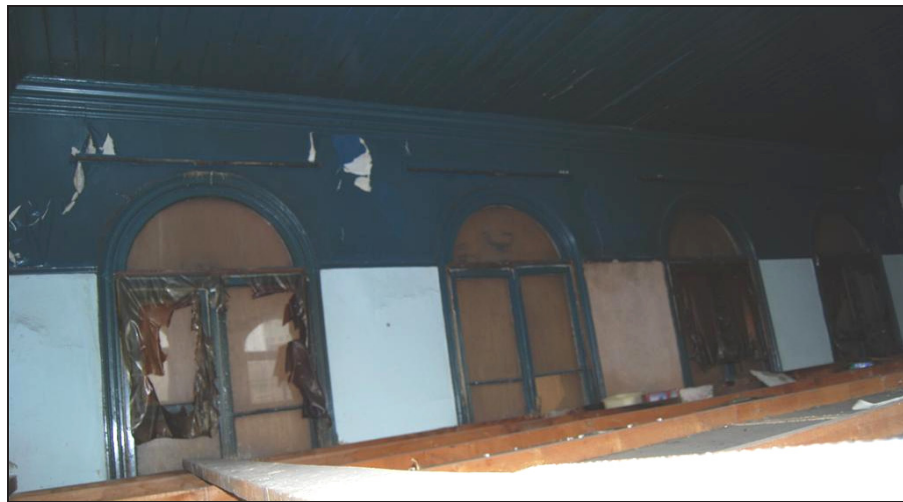
Plate 10: View Southwest above the Inserted Ceiling
