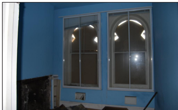
Plate 12: Room F3 looking northeast
