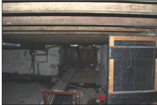
Plate 7: Room B1 Looking West to Barrel Hatch Doors
