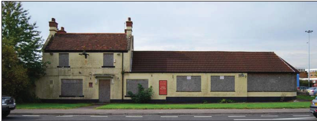
Plate 4: Northern Elevation, the Swan Inn
