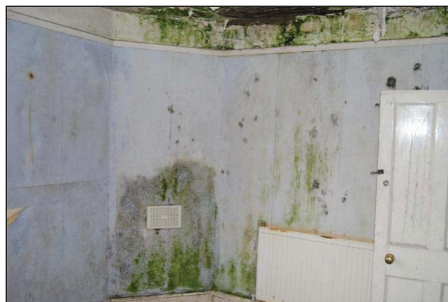
Plate 7: Room F6 looking North
