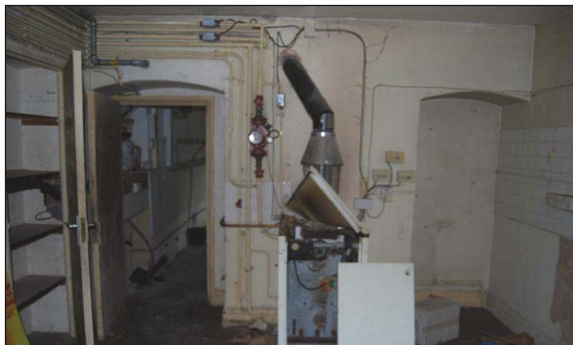
Plate 10: Room G9 looking North
