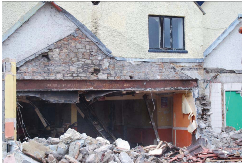
Plate 6: Roof scar behind extensions
