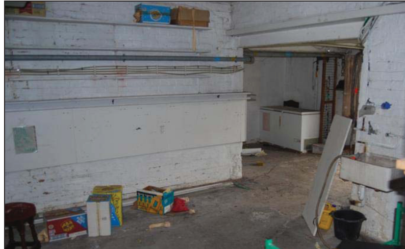
Plate 14: Barrel store (Room G10) looking Northwest
