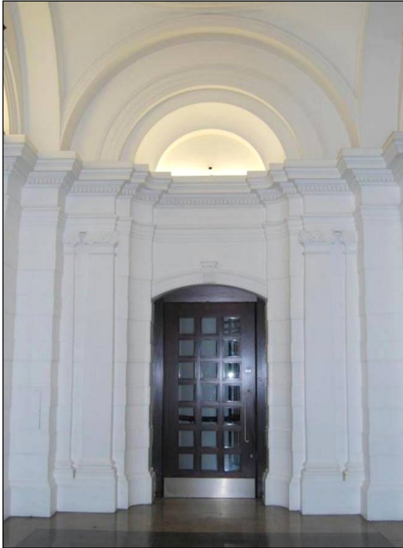
Plate 6: Door Type B to Spiral Staircase.
