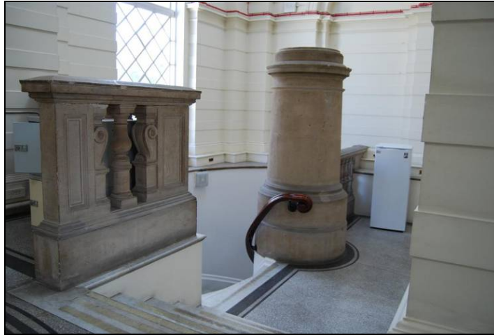
Plate 7: Newel Post and Masonry at top of Spiral Stair
