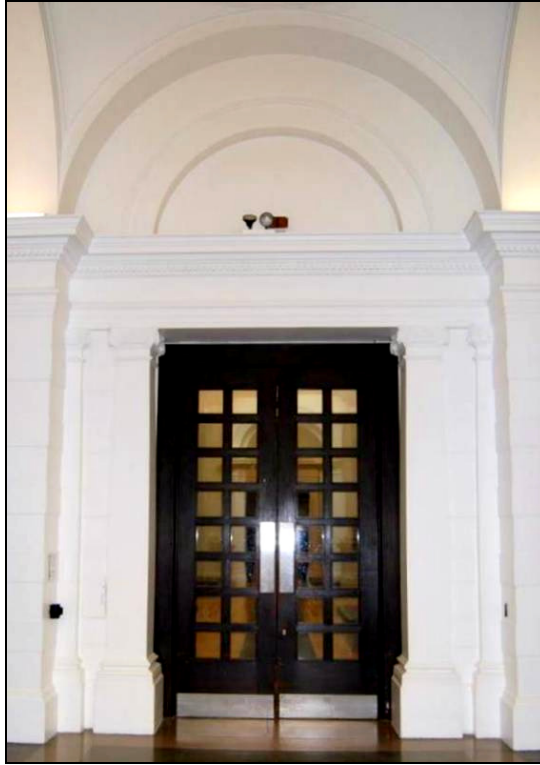
Plate 5: Door Type A to Gallery 1, Looking South
