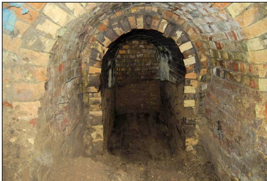
Plate 55: Blocked Flue
