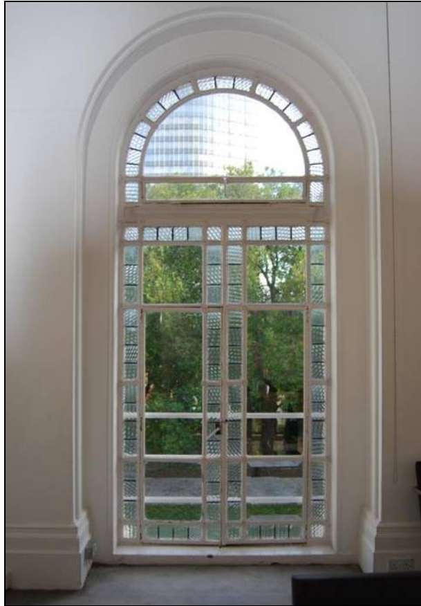
Plate 17: Meeting Room Window, looking East
