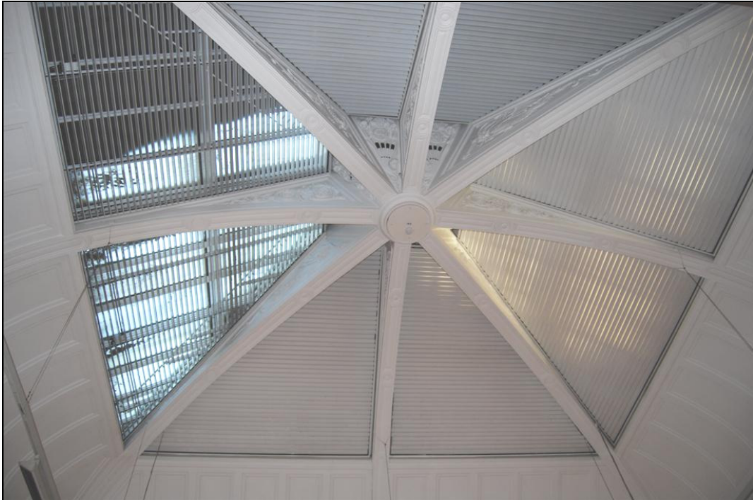
Plate 27: Overview of Roof Assembly, Room T8P.32
