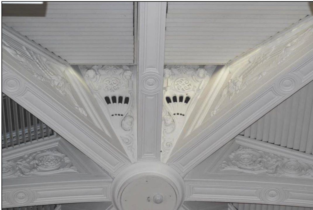
Plate 28: Detail of Moulded Decoration, Roof Trusses, Room T8P.32
