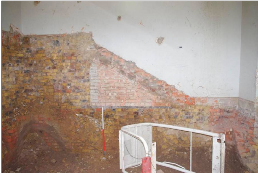
Plate 11: Stairs Removed below Ervin Bossanyi Stained Glass Window
