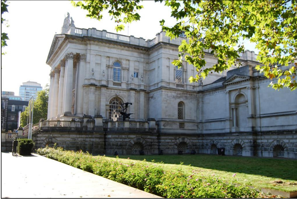
Plate 47: Northern Part of Eastern Elevation and Portico
