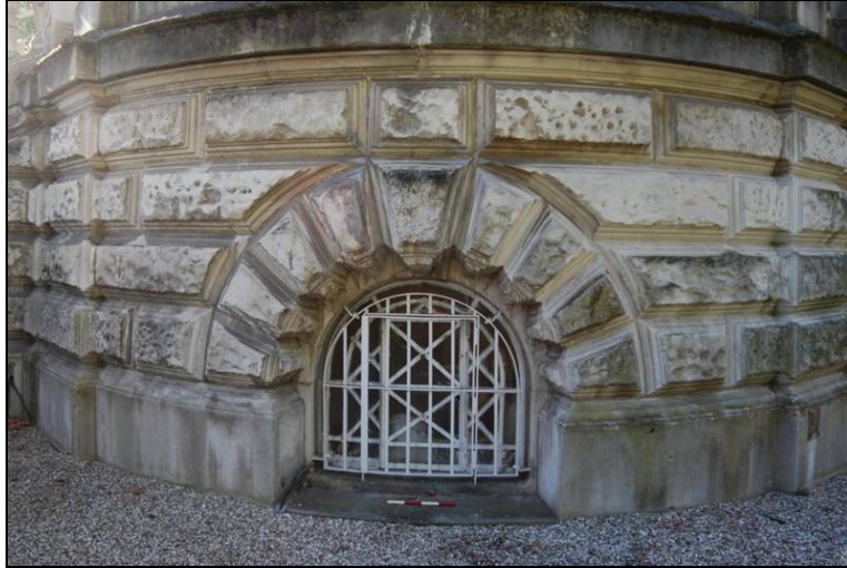
Plate 49: Window Detail to Room T1G.16.1 Type D
