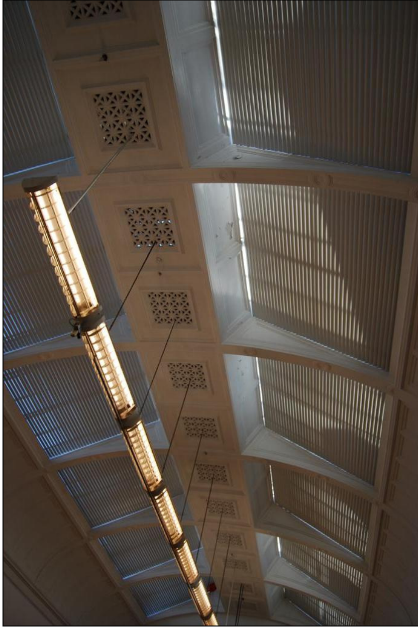
Plate 30; Roof structure of Gallery 35
