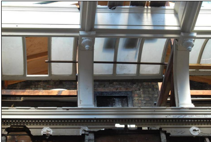
Plate 22: Turned Finials on ceiling structure. Upper floor.
