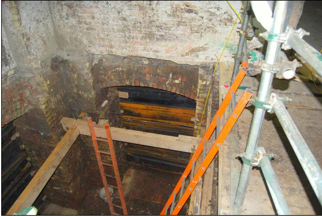
Plate 53: Excavation of Trench 4
