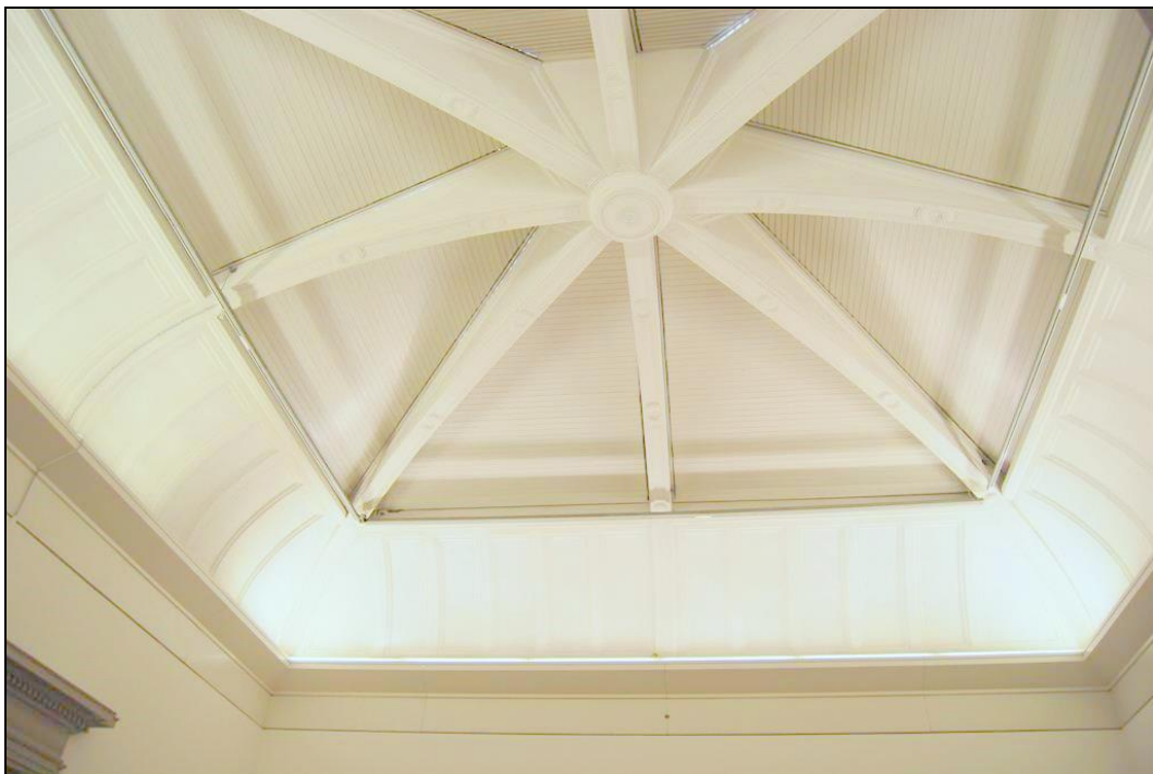
Plate 40: Gallery 39, Roof Detail
