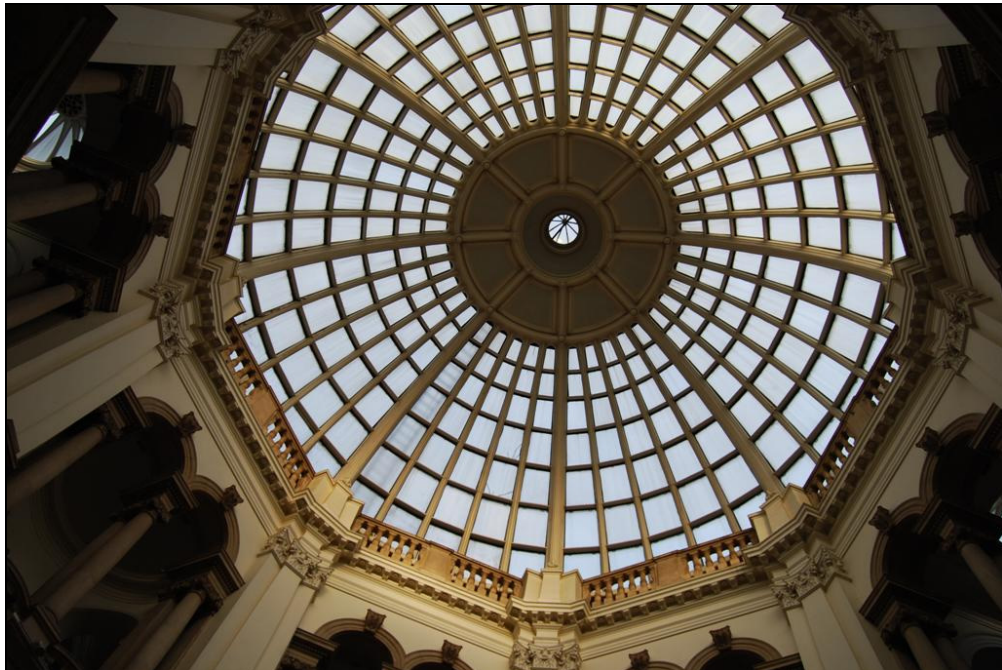
Plate 13: Dome Above Rotunda
