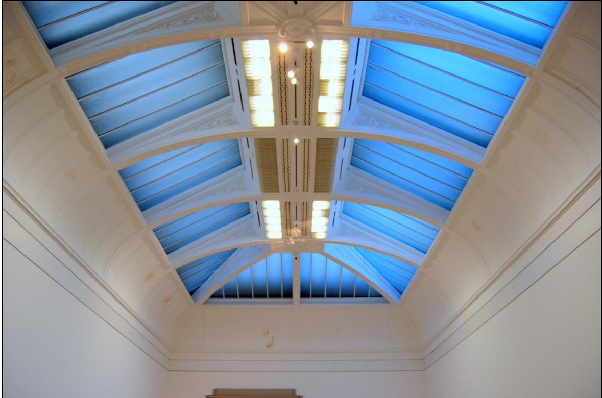
Plate 29: Roof assembly, Room T8P.33
