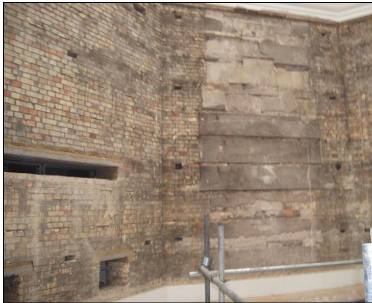
Plate 23: Stone Blocks Form the Rear of the Arched Recesses, Room T8P.31
