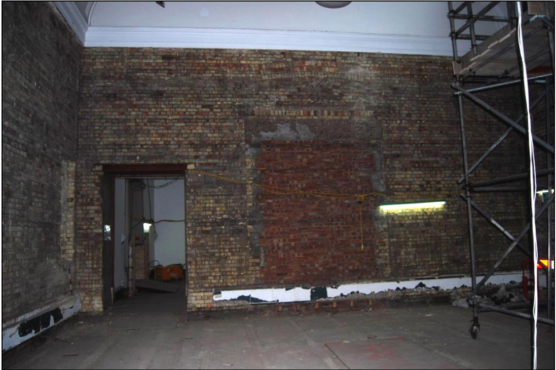
Plate 35: Original Doorway , North Wall of Gallery 36
