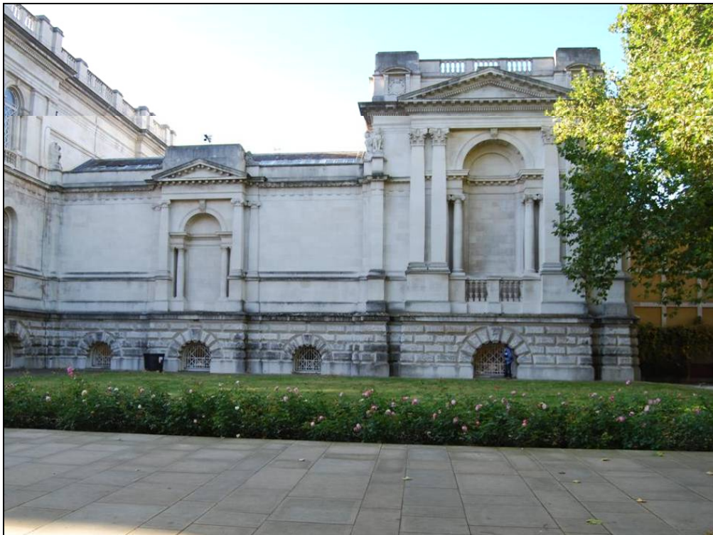
Plate 48: Northern Part of Eastern Elevation
