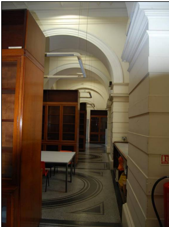
Plate 15: Rotunda Upper Level looking West along the South side
