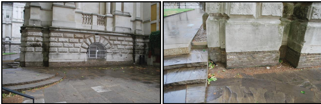
PLATE K & L: View showing the area of previous ground reductions to the north of the proposed area of external development (left) and view showing exposed brick footings of the Tate building and the difference in height between the two areas.
