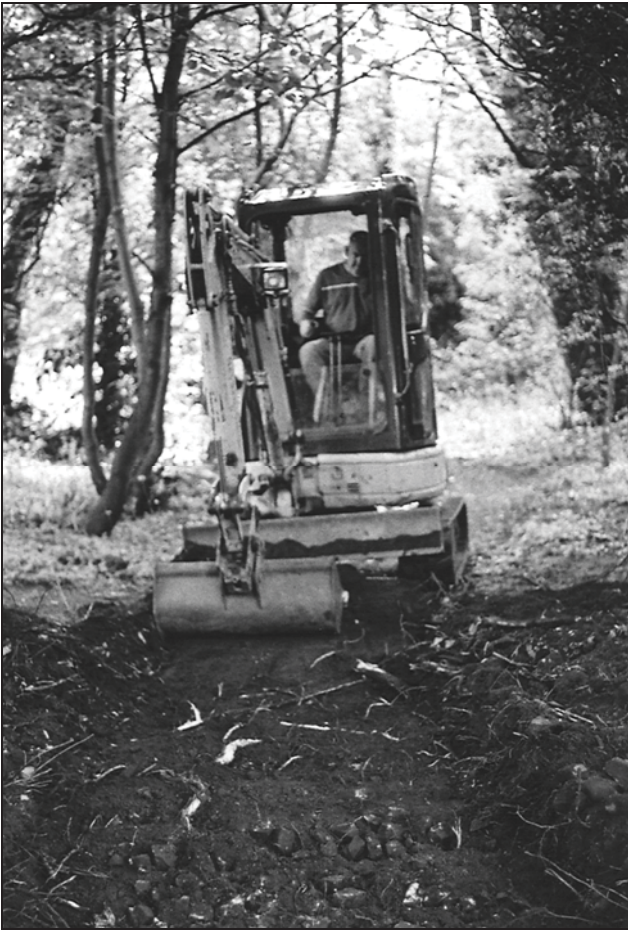
Plate 1: View of excavation of path from south-west
