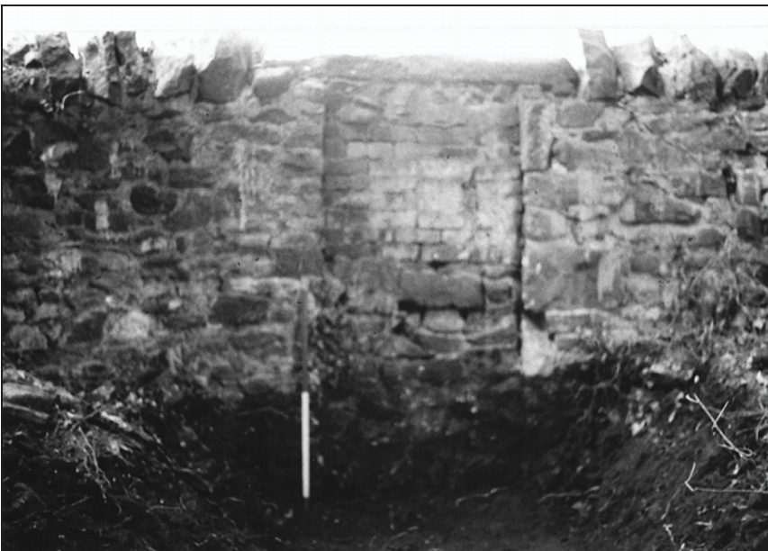
Plate 2: Blocked opening from north-east
