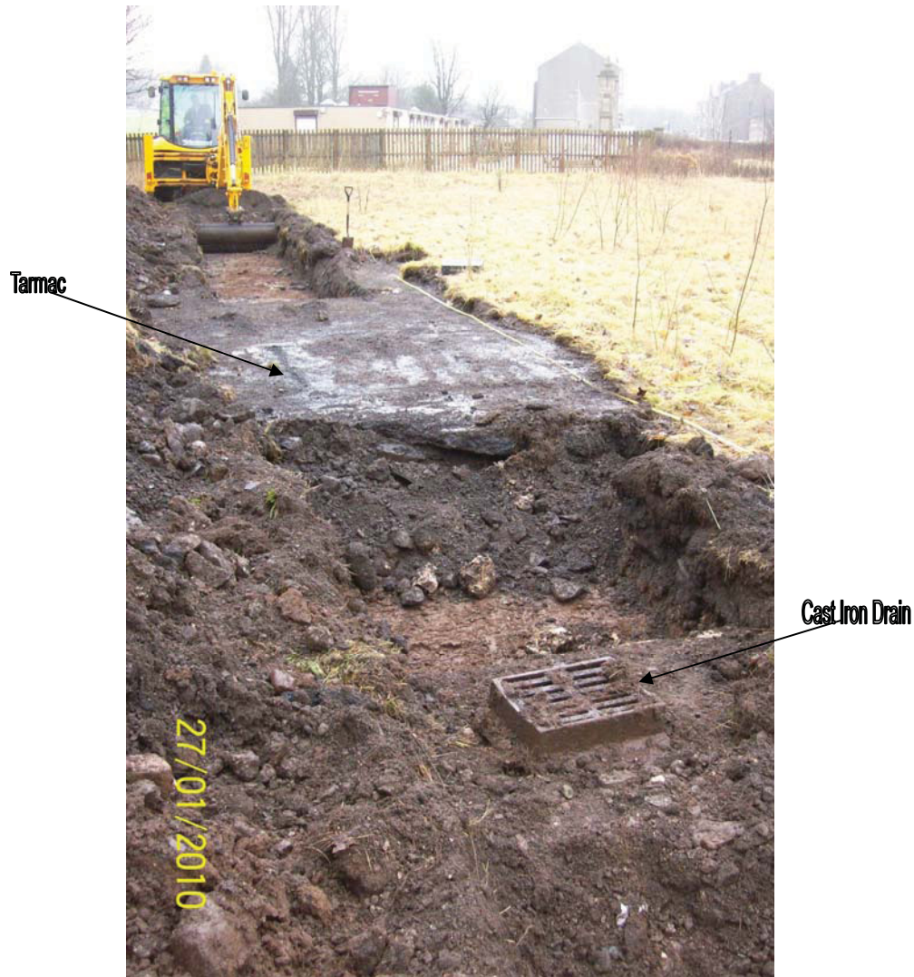
Plate 1: Trench 1 showing cast iron drain and tarmac
