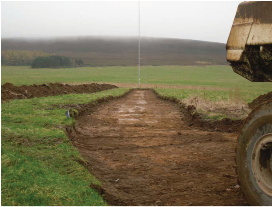
Plate 2: Topsoil stripped access track
