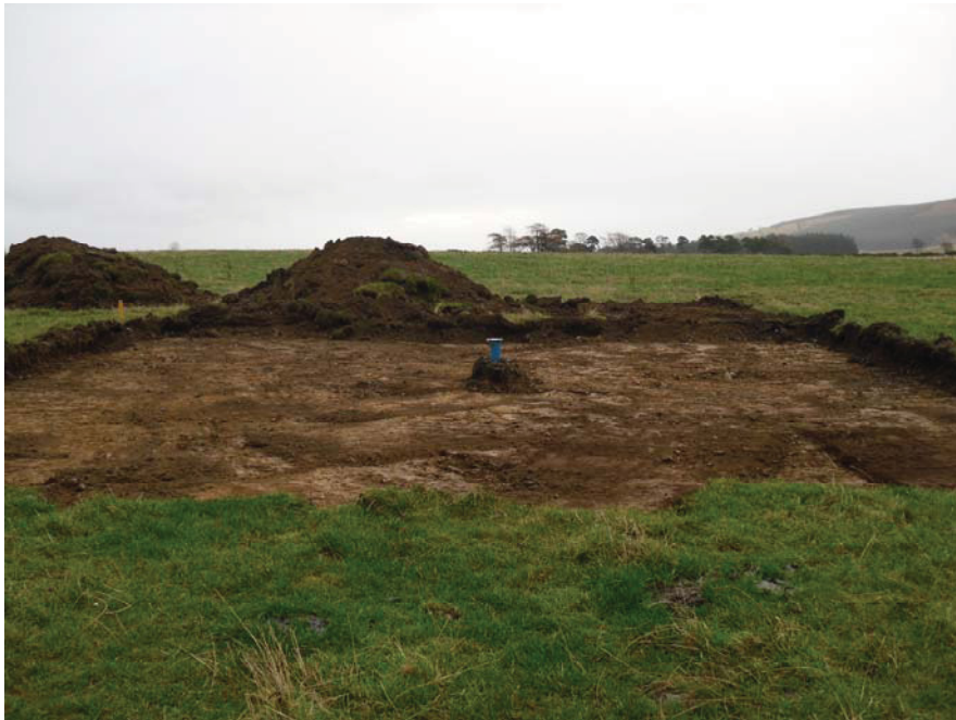
Plate 1: Topsoil stripped hardstanding area
