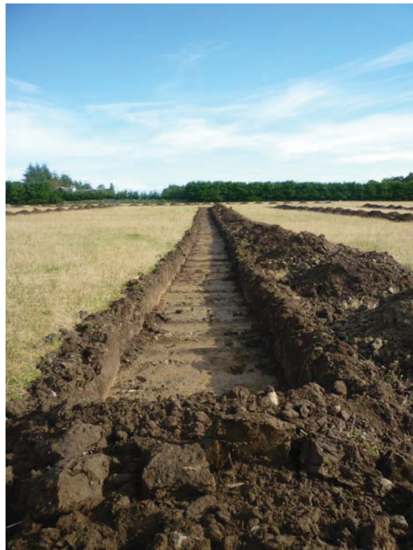
Plate 1: Trench 27 from south
