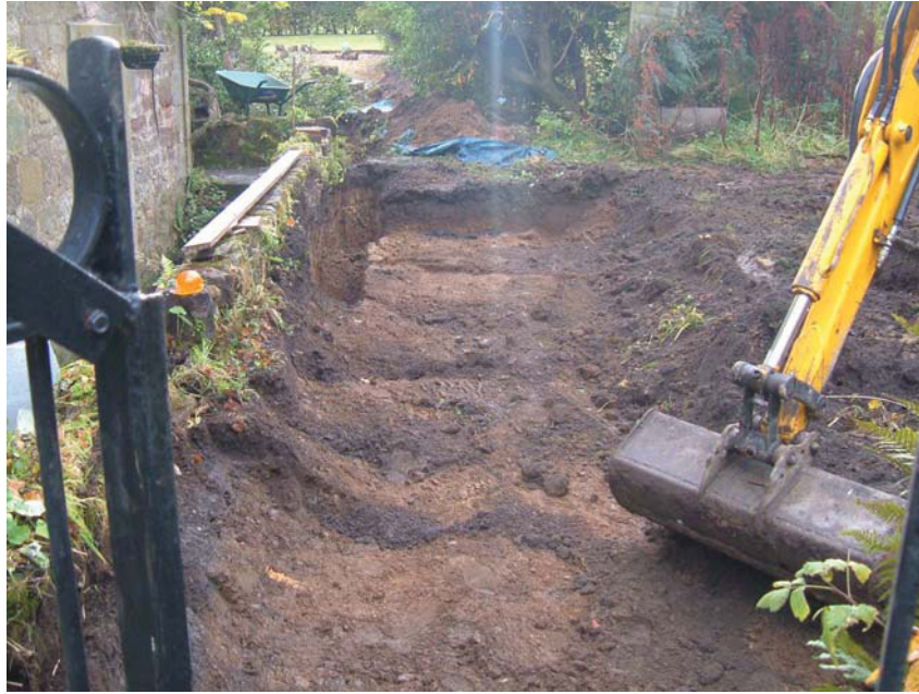
Plate 2: Working shot of area under excavation
