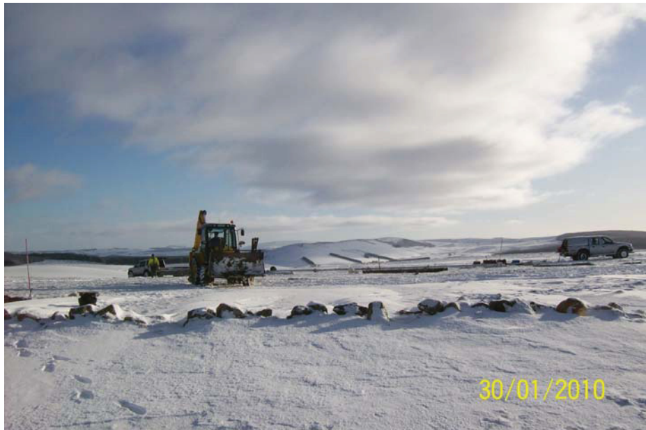
Plate 2: General view across working site from North
