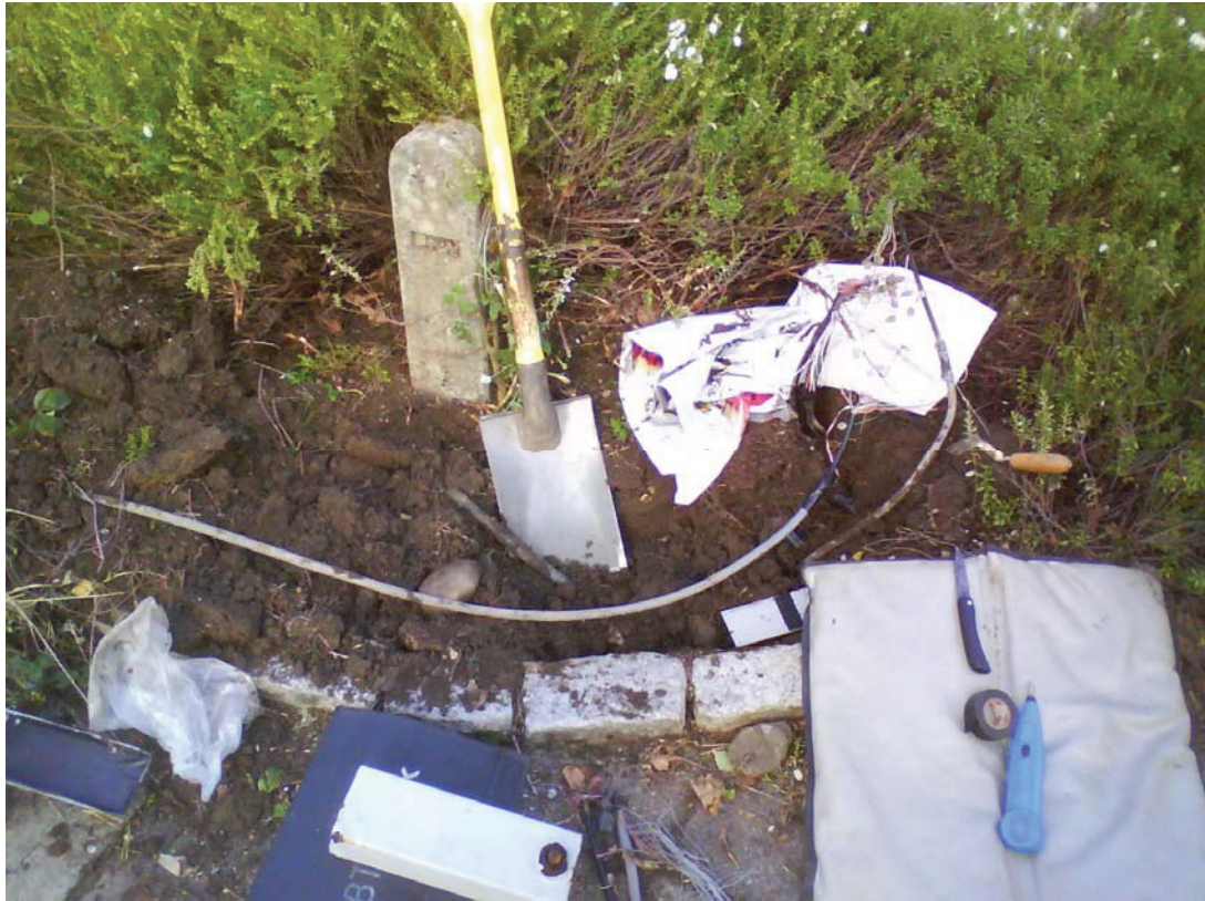
Plate 1 Showing existing apparatus exposed and extent of ground disturbance
