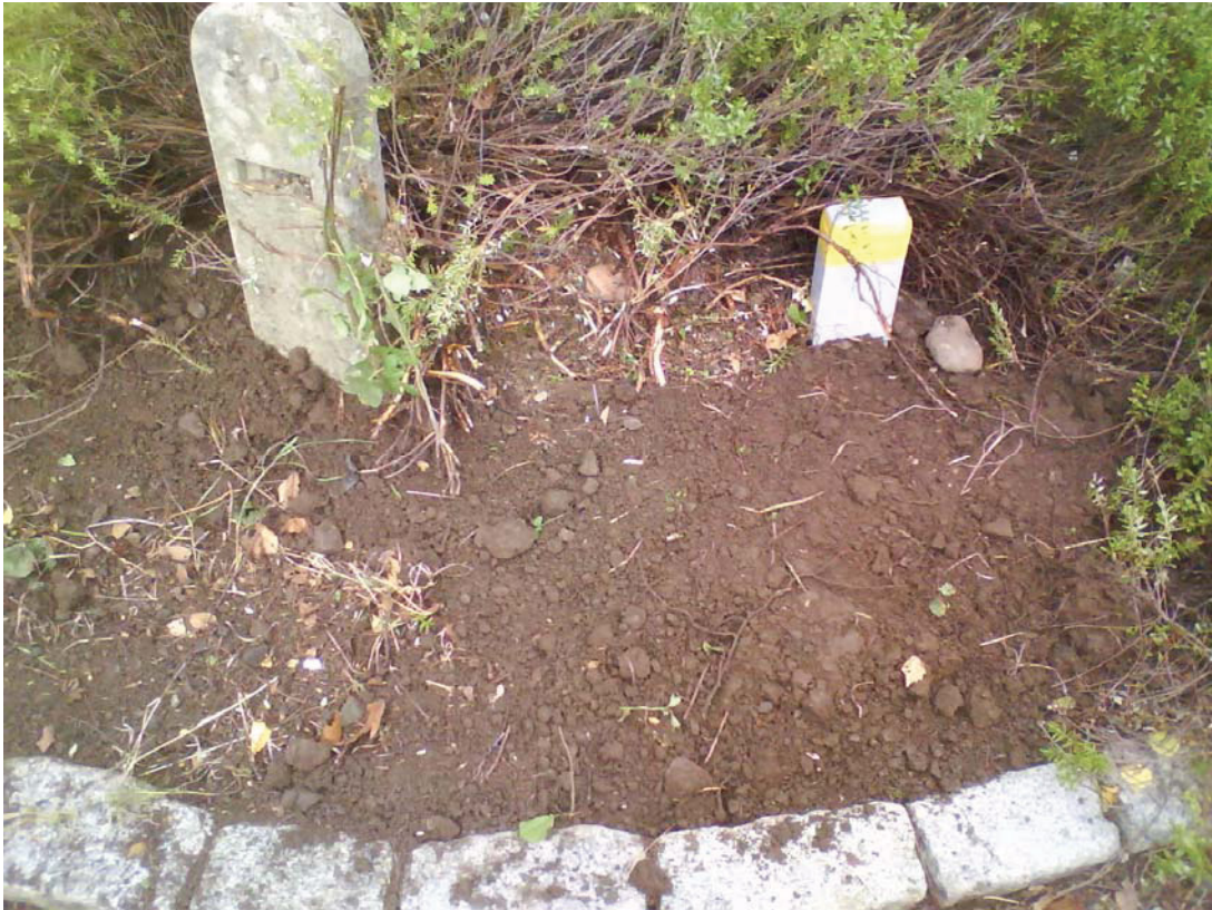
Plate 2 Showing excavations reinstated
