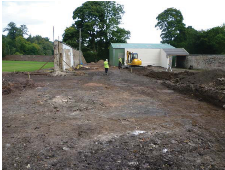
Plate 1: Working shot of area under excavation
