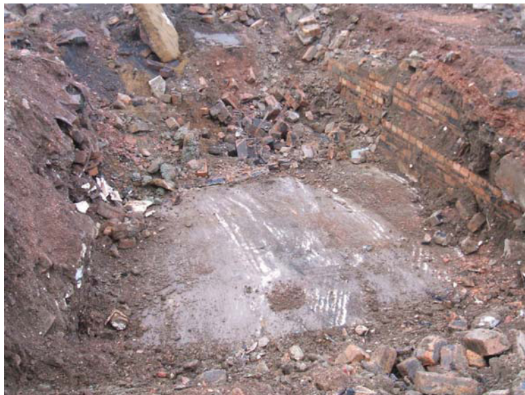
Plate 2: Concrete floor at base of topsoil strip
