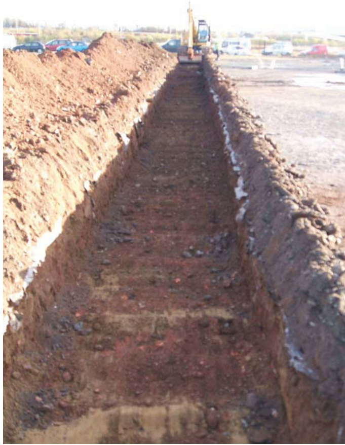
Plate 3: Post-excavation shot of Trench 2
