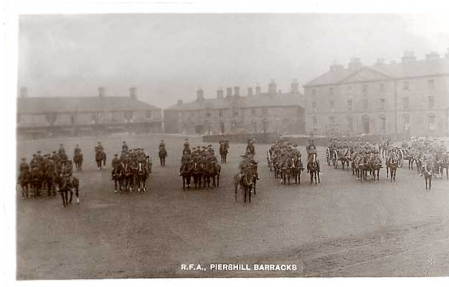
Plate 1: Detail of Piershill Cavalry Barracks
