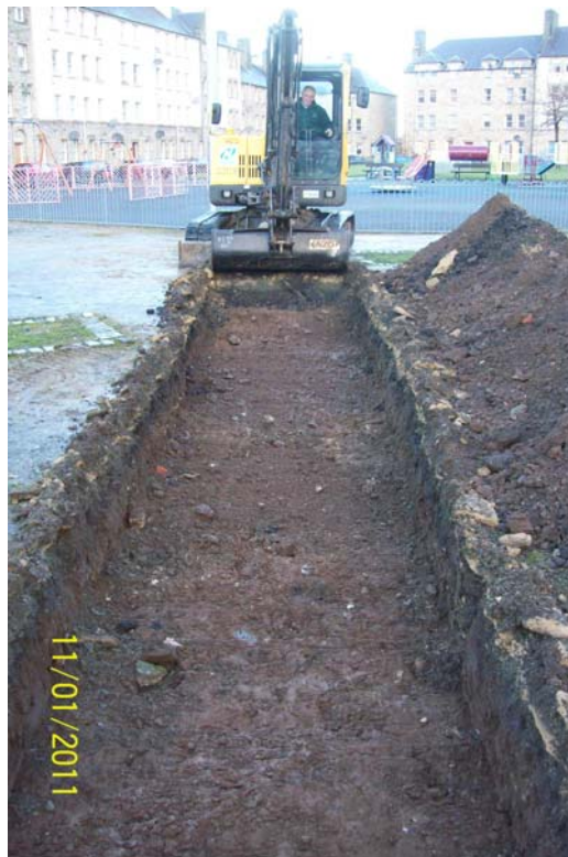
Plate 3: Detail of Trench 2
