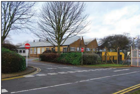
Plate 19: Building 10/8 Looking Northwest.
