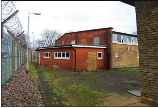
Plate 21: West End of Building 10/8 Looking North.
