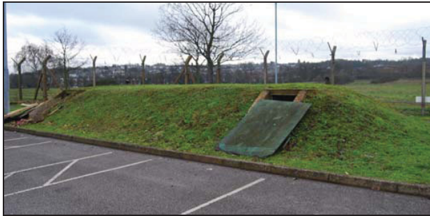
Plate 1: View of Eastern Air Riad Shelter
