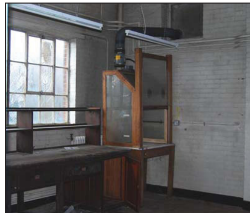
Plate 13: Chemical Laboratory Looking Northwest, Internal.
