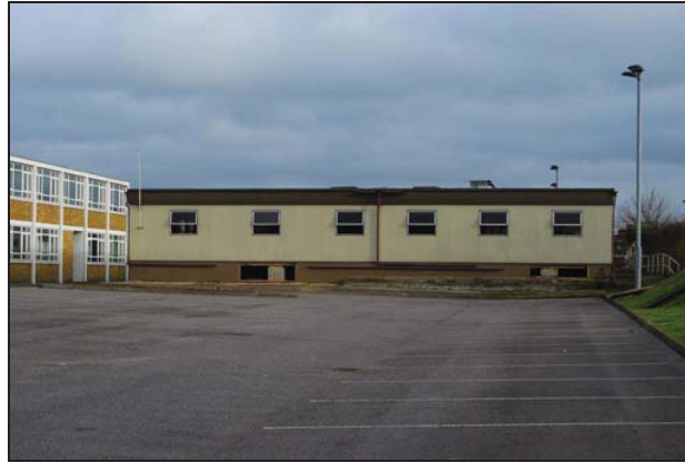
Plate 25: Building 10/12 Looking East
