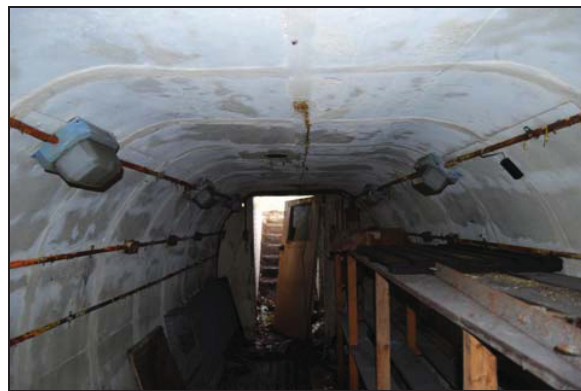
Plate 9: Western Shelter, Looking East
