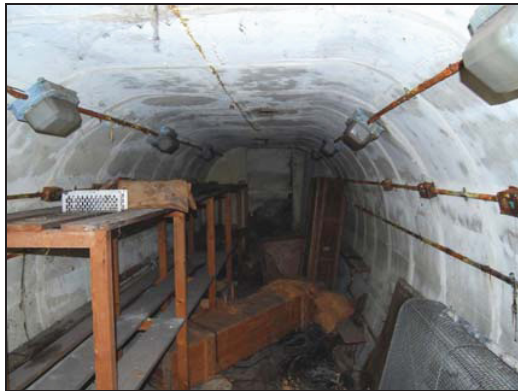
Plate 8: Western Shelter, Looking West
