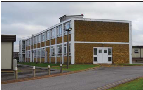
Plate 23: Building 10/10 Looking Southeast.
