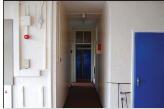
Plate 32: Building 10/15 Corridor Looking East.
