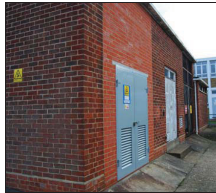
Plate 27: Building 10/13 Looking Southeast
