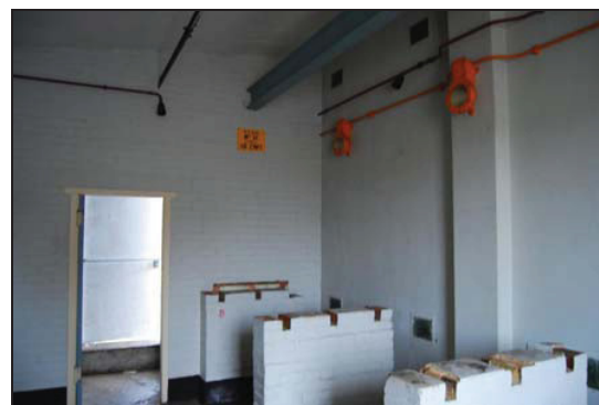
Plate 17: Internal View of Chemical Store.
