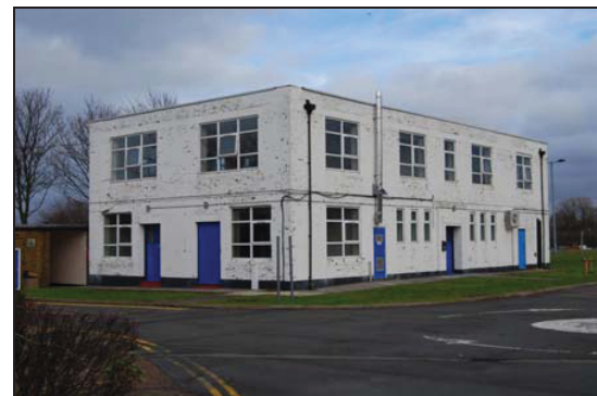
Plate 34: Building 10/17 Looking Northwest
