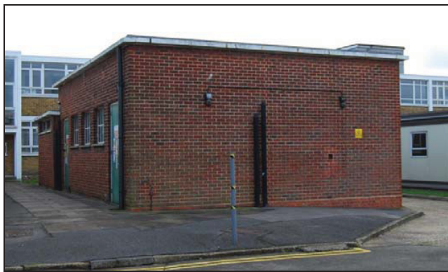
Plate 26: Building 10/13 Looking Southwest
