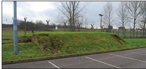
Plate 7: Western Bunker, Looking Southwest
