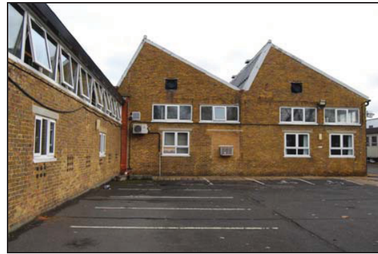
Plate 22: Building 10/8 Looking East
