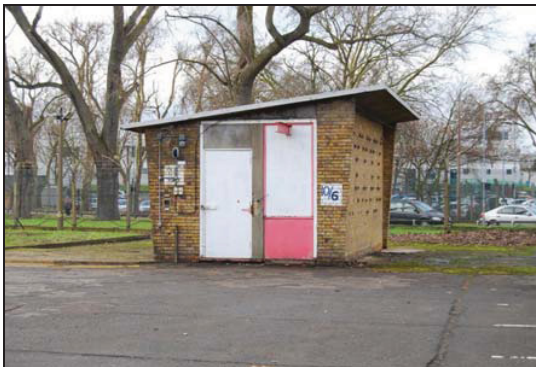
Plate 16: Chemical Store Looking West.
