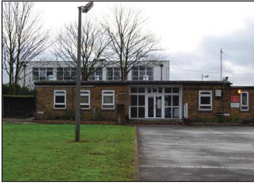
Plate 31: Front of Building 10/15, Looking South.
