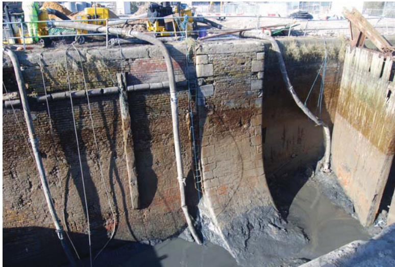
Plate B: Basin walling and buttress curving into base
