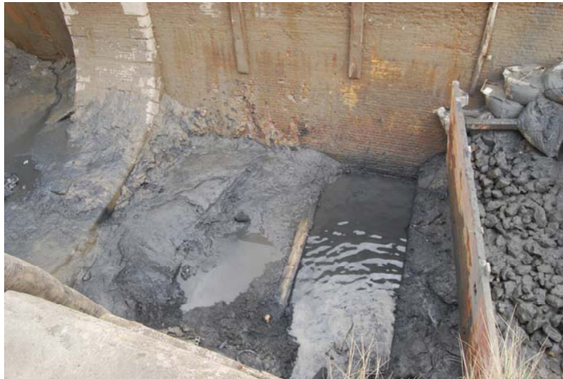
Plate C: Base of basin showing timber compartmentalisation
