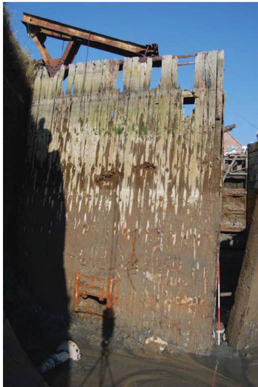
Plate H: Seaward face of outer lock gate showing planking and sluice
