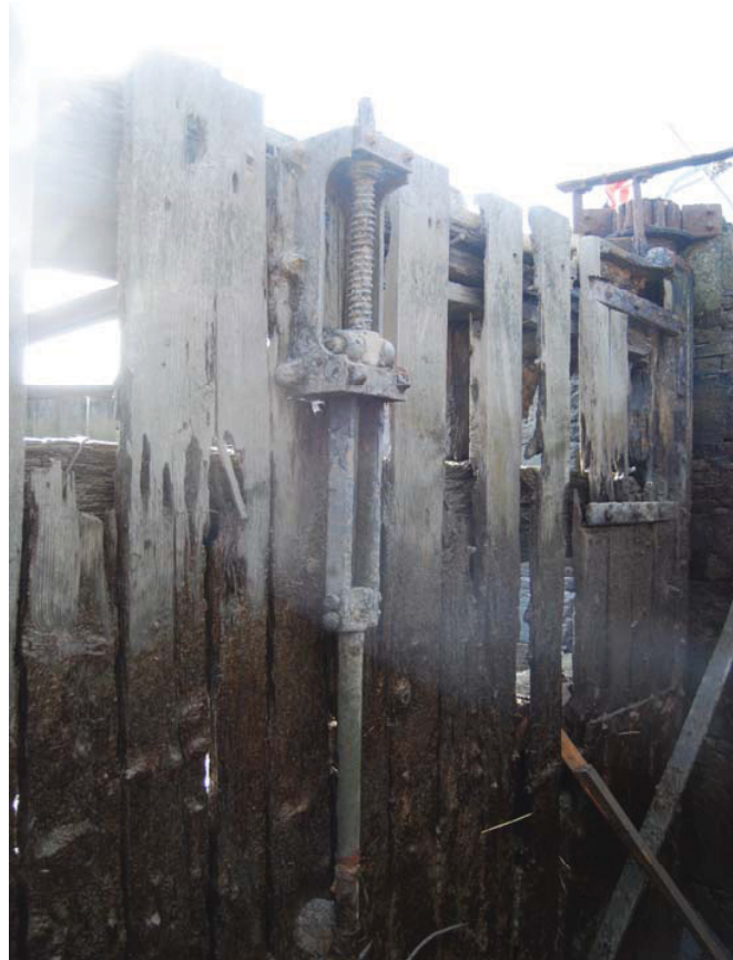
Plate F: Detail of sluice mechanism on inner lock gate
