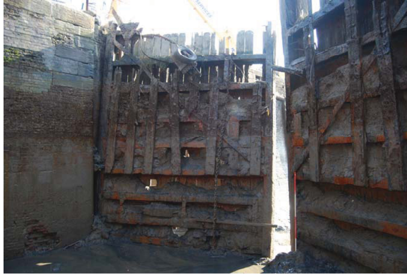
Plate G: Landward side of outer lock gates showing framing
