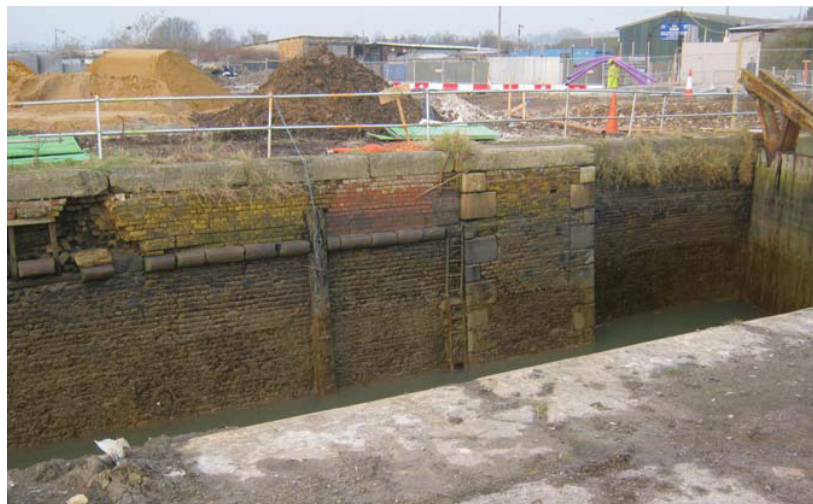
Plate D: Basin wall showing coping, rubbing fender and ladder
