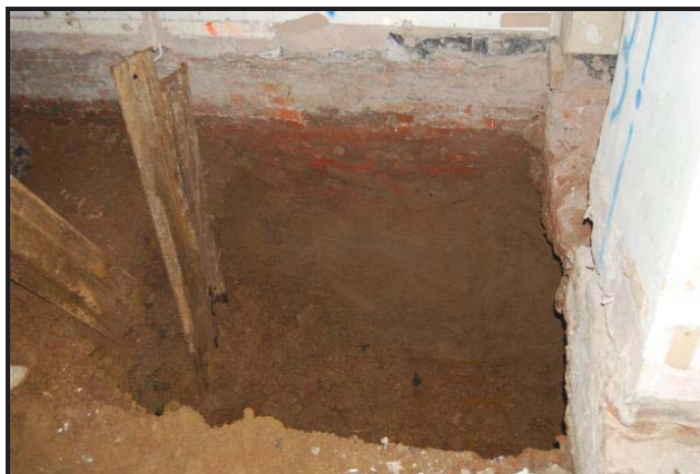
PLATE F: General shot of underpinning pit 7
