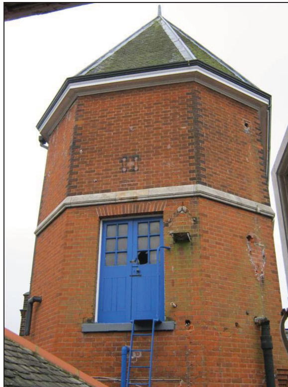
Plate 142: External Detail of Water Tower
