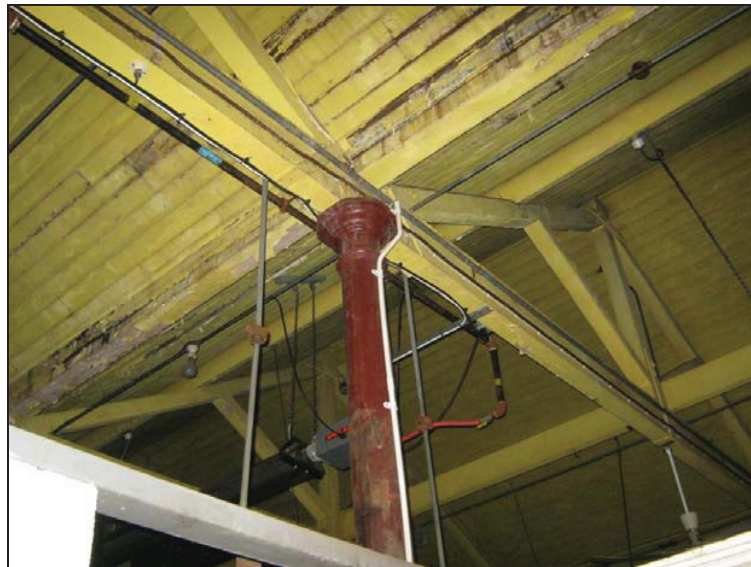
Plate 150: Roof Truss and Iron Column
