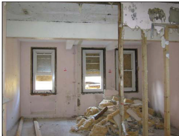
Plate 81: Room 8 Looking Southeast
