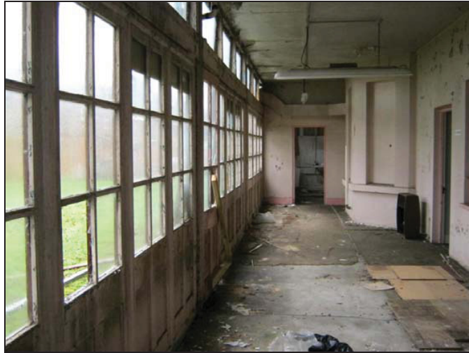
Plate 9: Ground Floor of Sun Ward, Looking Northwest
