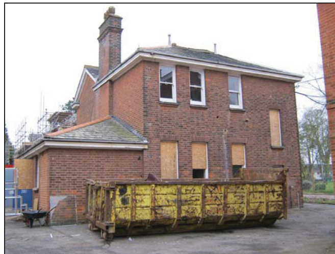
Plate 76: View Looking Southeast
