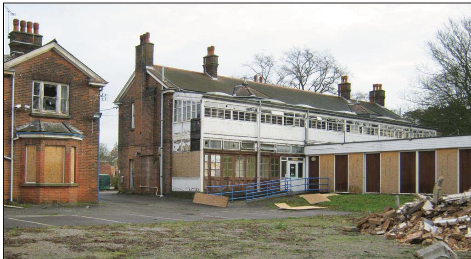
Plate 21: Rear of Building EHW 4, Looking East
