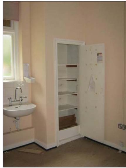
Plate 94: Room 20 with Original Cupboard
