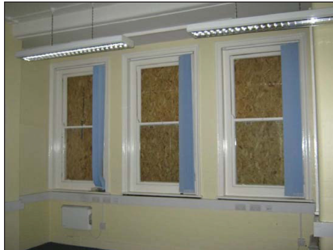
Plate 139 Room 44 Looking West
