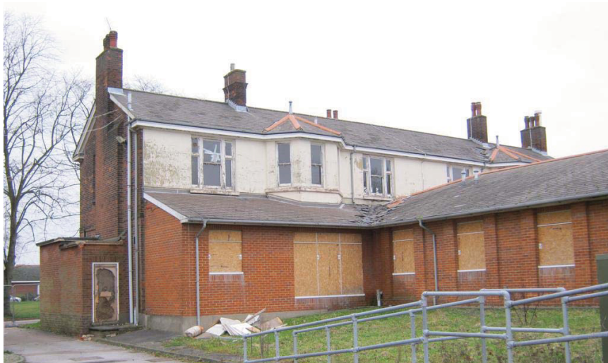
Plate 59: Rear of Building EHW 10
