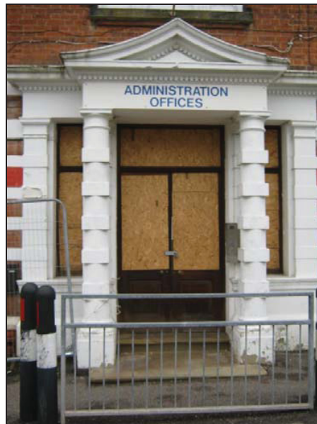
Plate 126: Detail of Main Entrance
