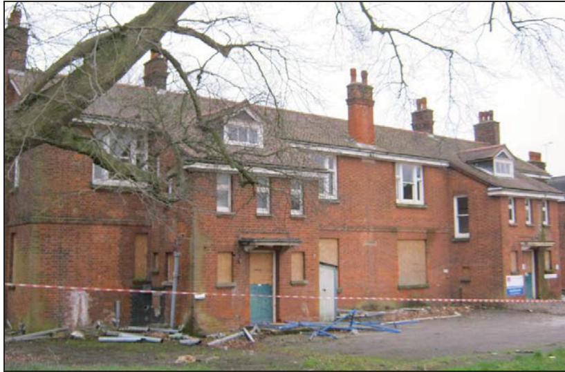
Plate 20: Building EHW 4, Looking West
