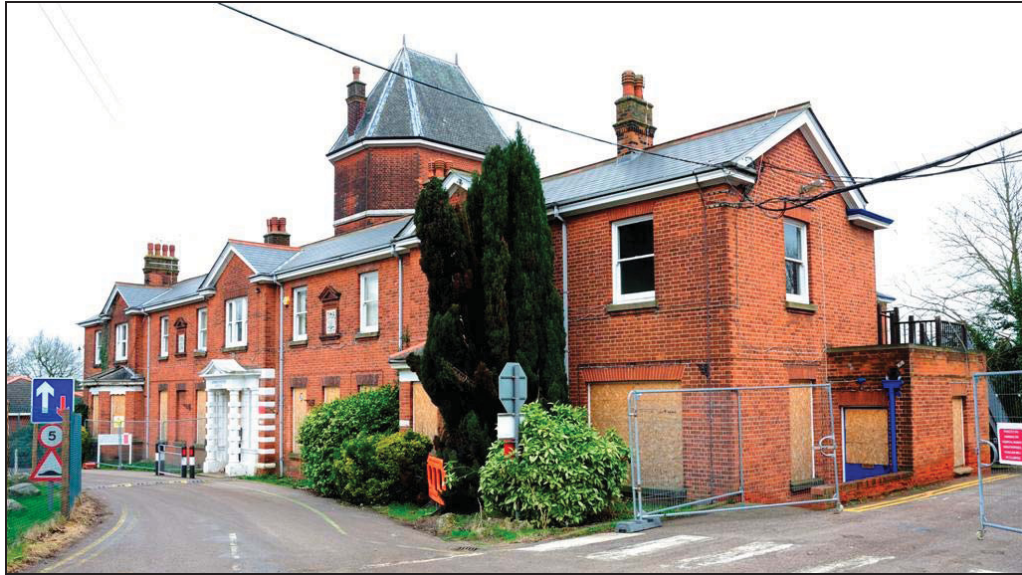
Plate 125: General View Looking North, EHW 22
