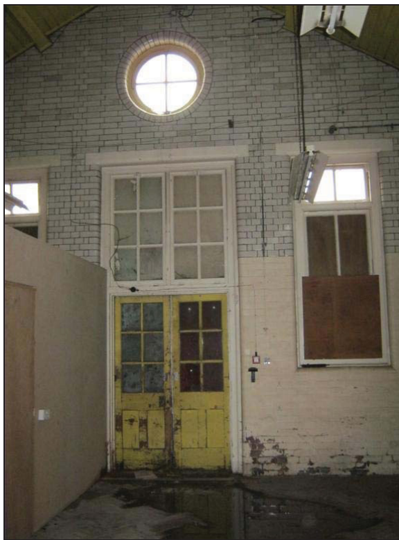
Plate 153: Room 2 Looking Southeast
