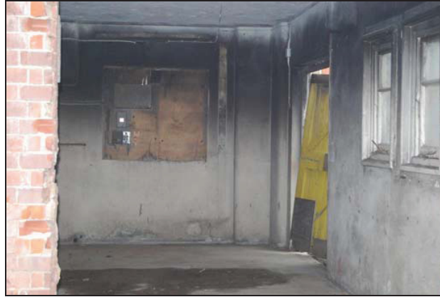
Plate 156: Room 2, Looking West
