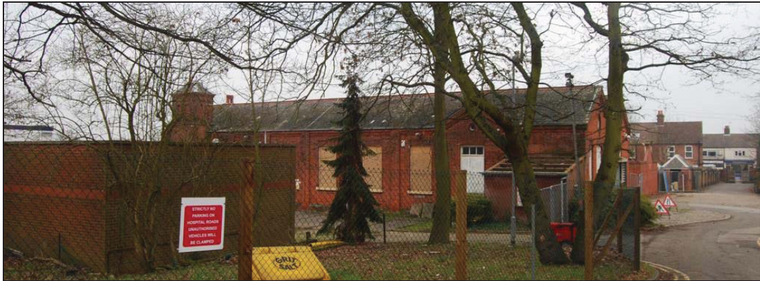
Plate 147: Building EHW 29 Looking North
