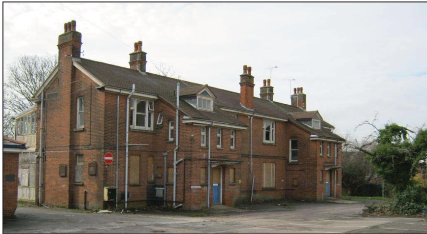
Plate 35: View of Building 6, Looking West
