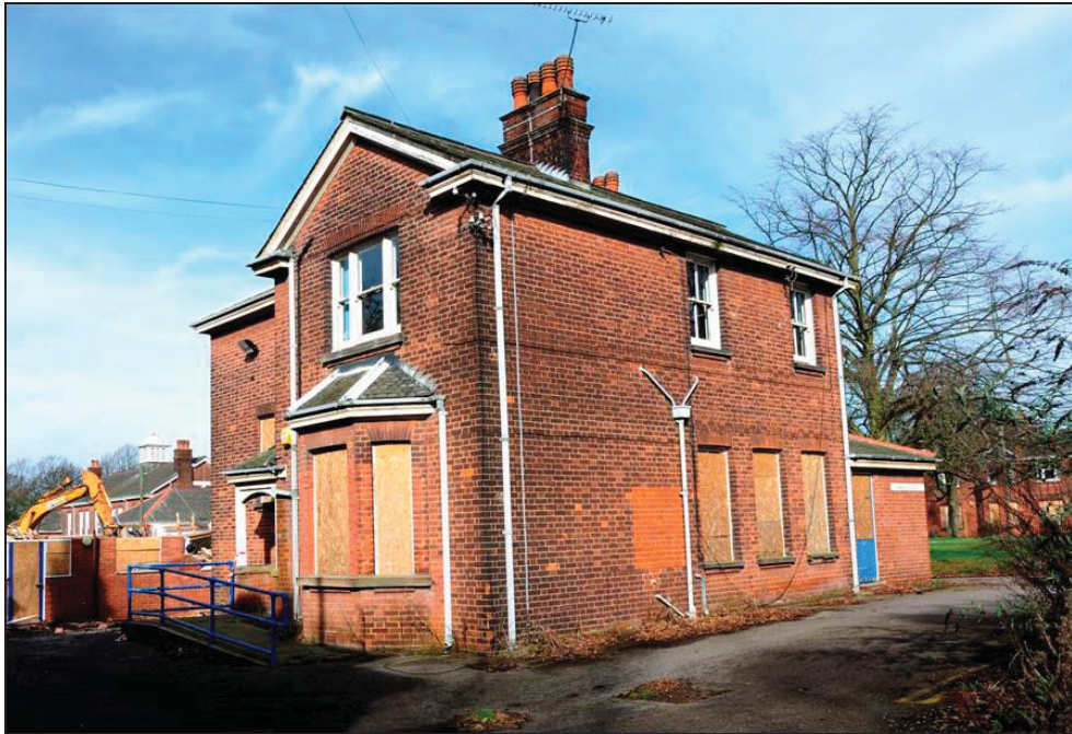
Plate 15: Building EHW 2 Looking North
