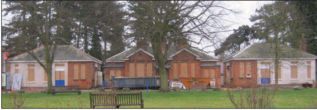
Plate 143: View of Building EHW 32, Looking Southeast
