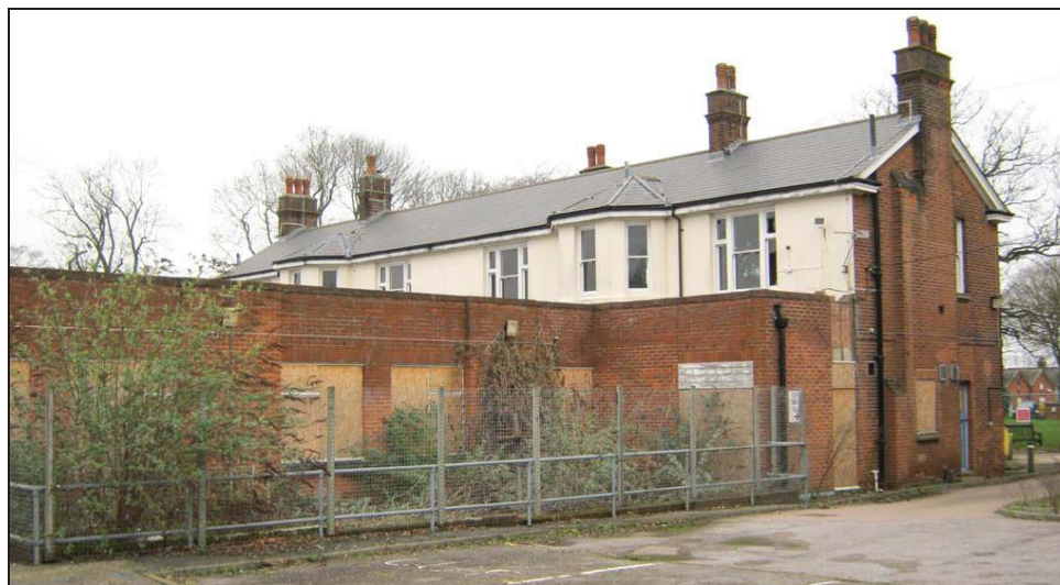
Plate 46: Building EHW 8 Looking North
