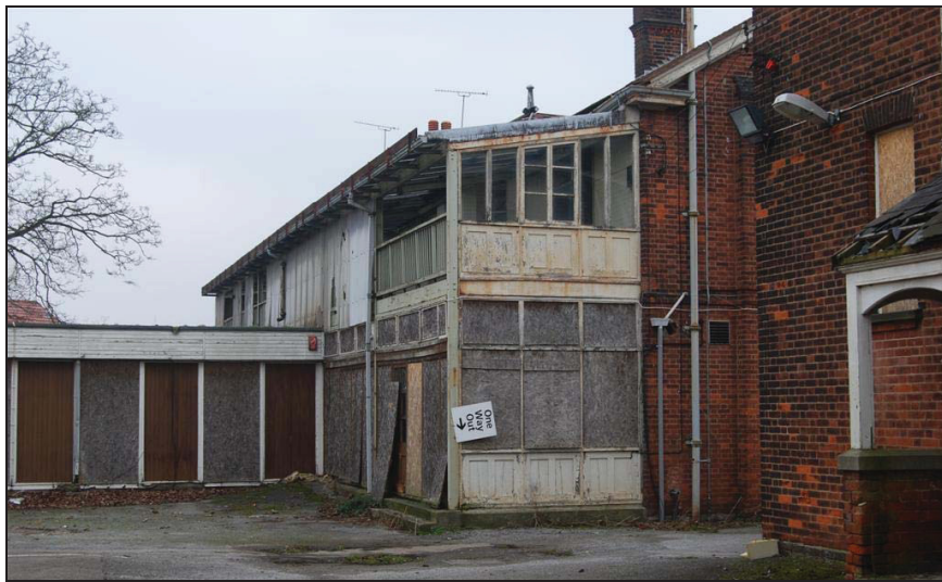
Plate 36: View of Building 6, Looking North
