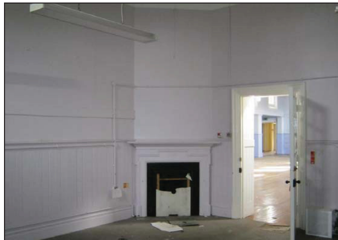
Plate 121: Room 1 Looking East
