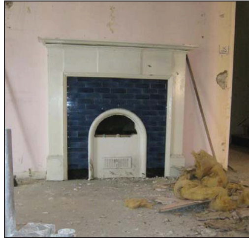
Plate 80: Room 3 Looking Southwest
