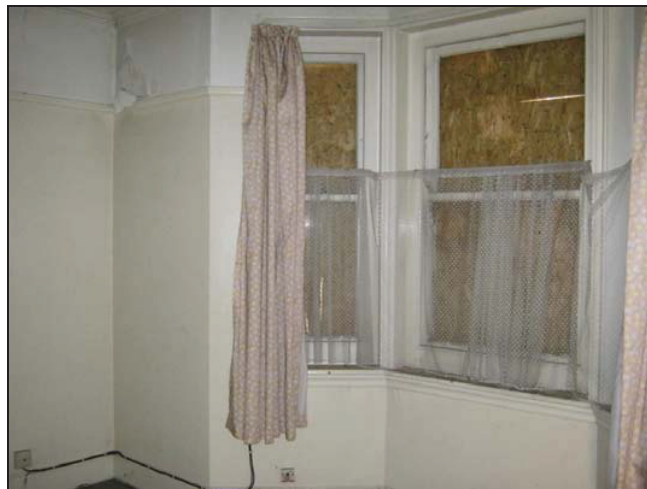
Plate 30: Room 4, Bay Window
