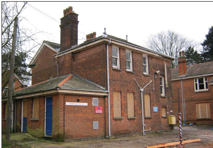
Plate 16: Building EHW 2 Looking South
