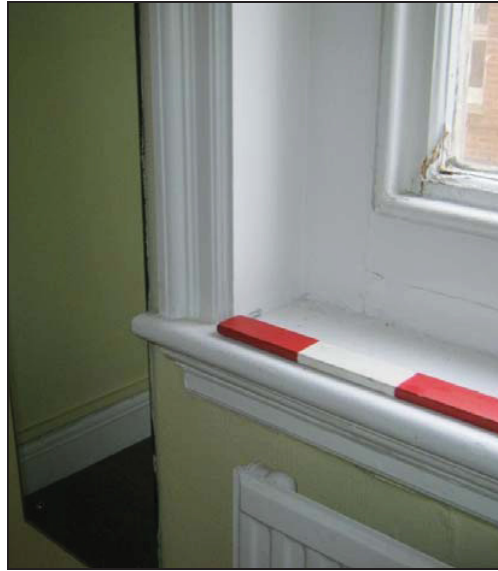
Plate 3: Typical Window Frame and Sill Moulding
