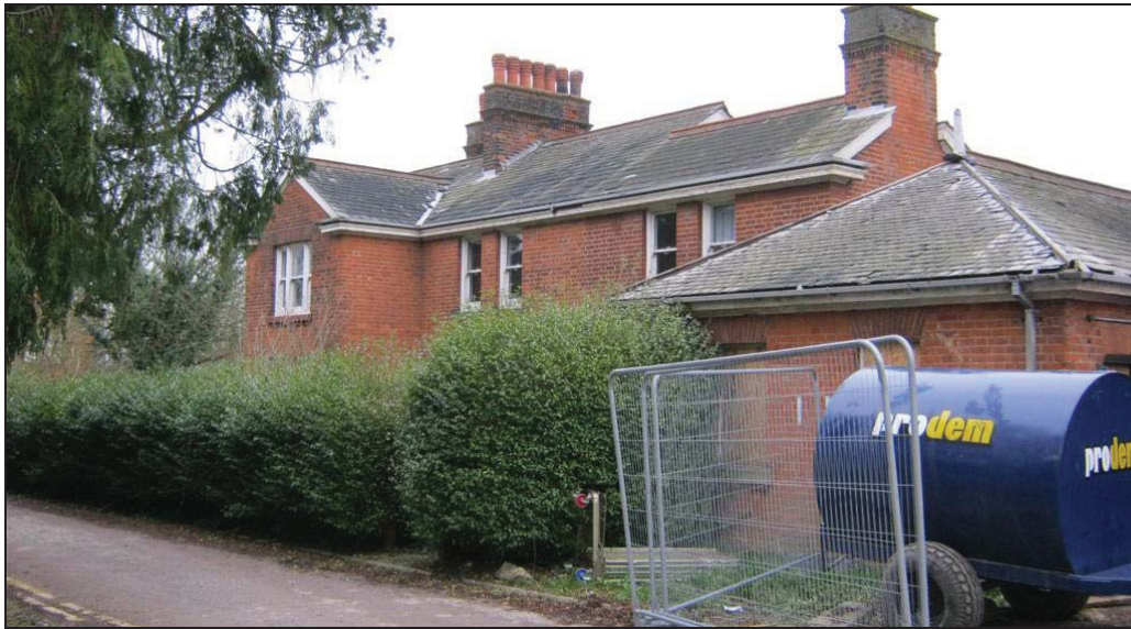
Plate 98; View Looking North
