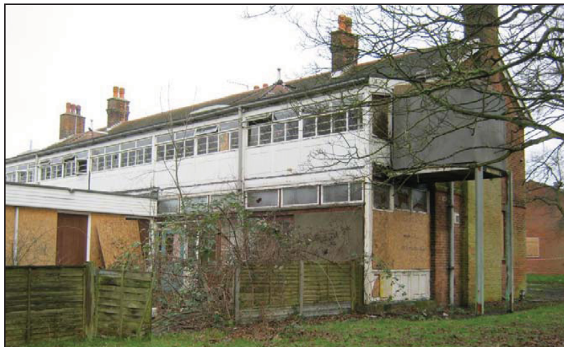
Plate 22: Rear of Building EHW 4, Looking North
