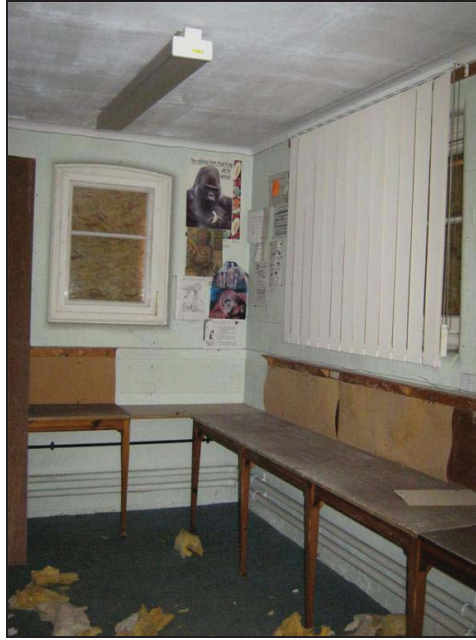
Plate 118 Room 12 Looking East
