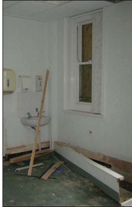
Plate 18: Room 8 Looking West
