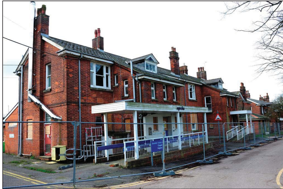
Plate 45: Building EHW 8 Looking West
