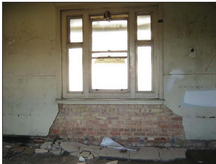
Plate 40: Sash Window of Central Ward
