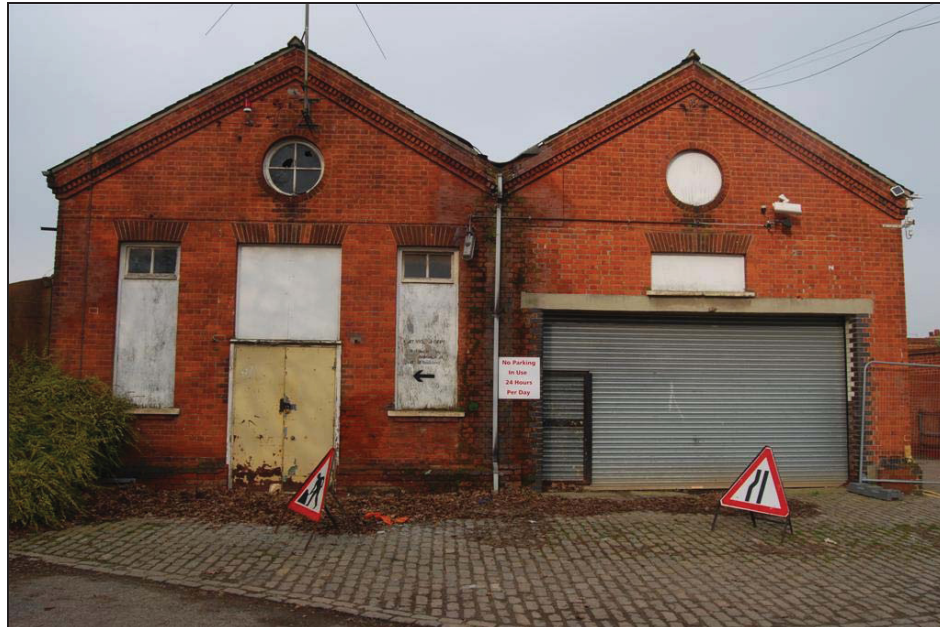
Plate 148: Building EHW 29 Looking Northwest
