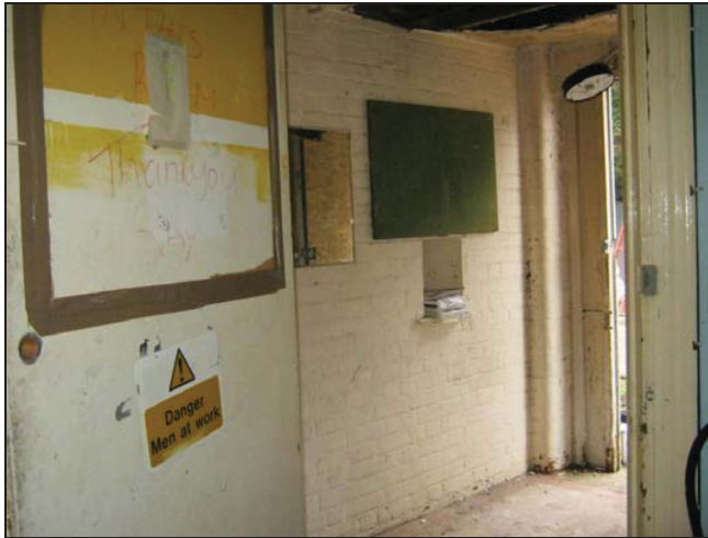
Plate 109: Entrance Hall with Hatch
