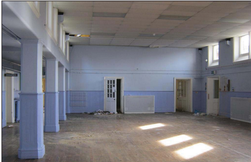
Plate 120: Room 8 Looking Southeast
