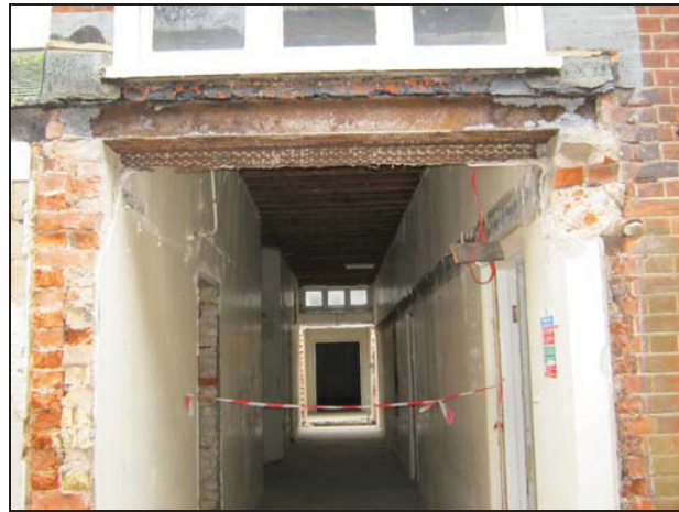
Plate 145: Steel Beam Across Join to Link
