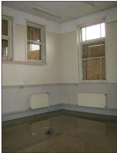
Plate 116: Room 18 Looking West
