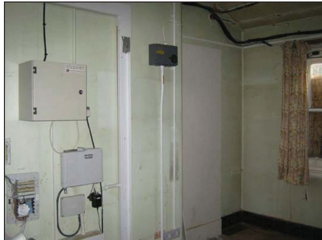
Plate 113: Room 13 Looking west
