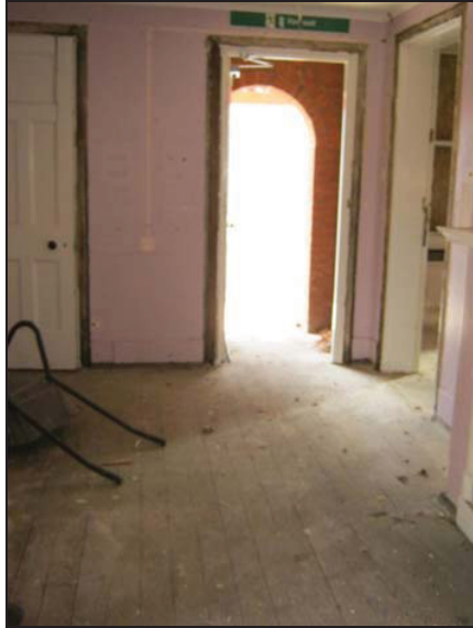
Plate 79: Room 2 Looking Southeast
