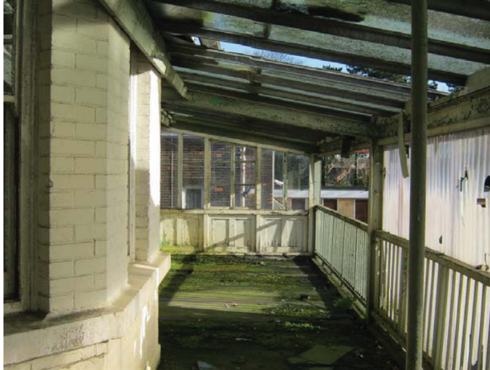
Plate 42: Room 45, Sun Ward Looking Southeast on First Floor
