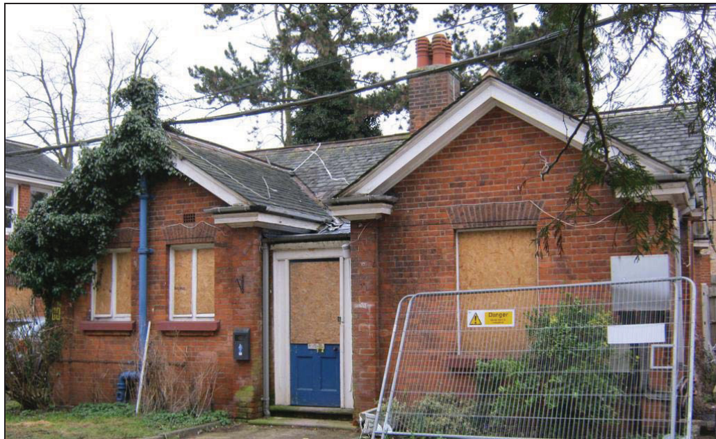
Plate 108: View Looking East of EHW 14
