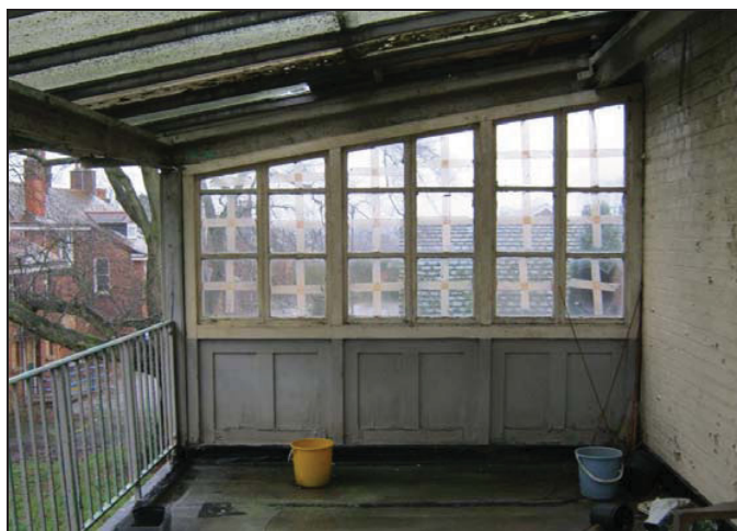
Plate 11: First Floor of Sun Ward, Looking Northwest
