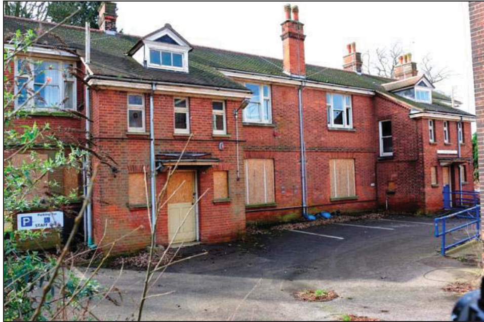
Plate 7: Building EHW 1 Looking West
