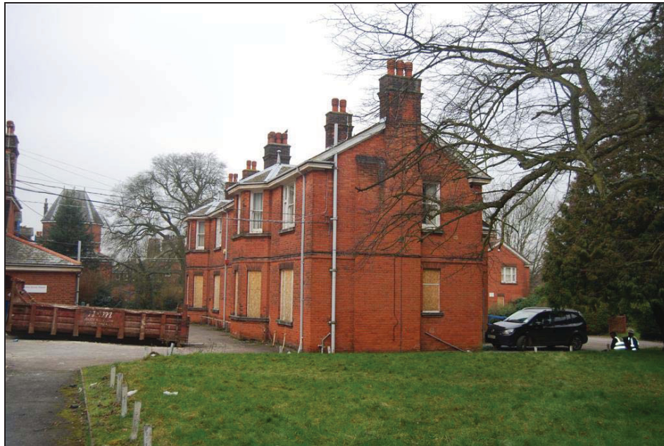
Plate 92: View looking North of EHW 19
