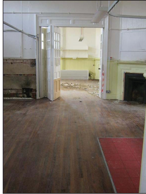
Plate 123: Room 9 Looking Southeast
