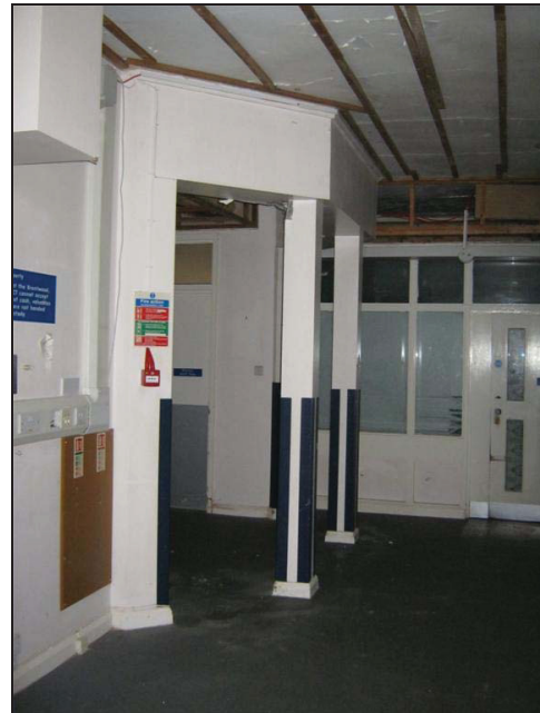
Plate 62: Demolished Bay Window
