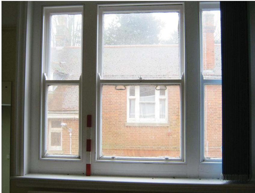
Plate 19: Sash Window, First Floor
