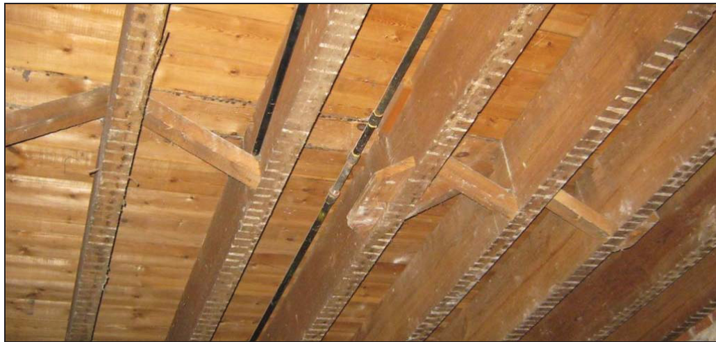
Plate 72: Room 17 Joist Braces
