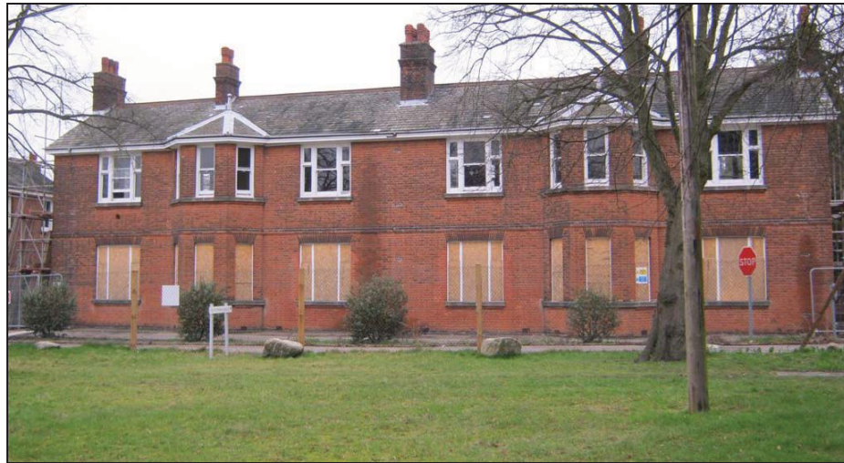
Plate 66: Building EHW 16 Looking Northeast
