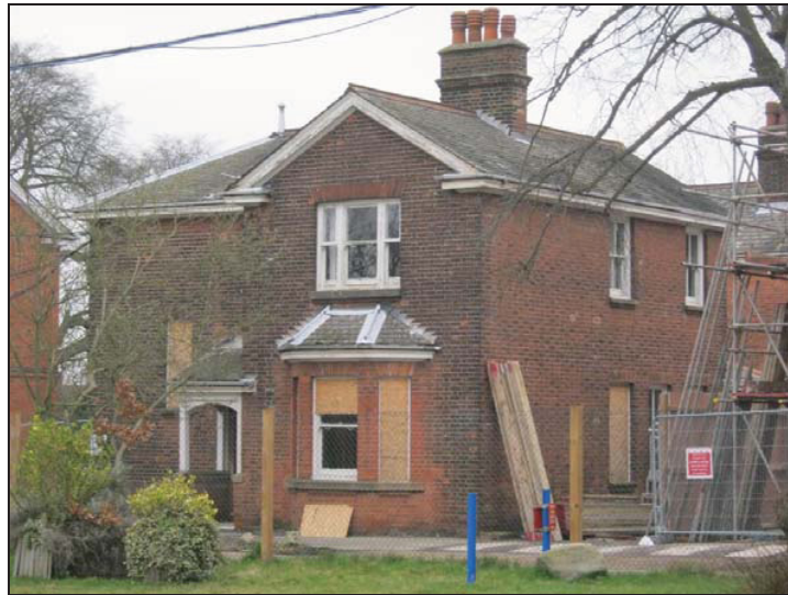
Plate 75: View Looking North of EHW 17
