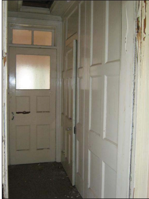
Plate 63: Original Panelled Cupboards, Door and Fanlight
