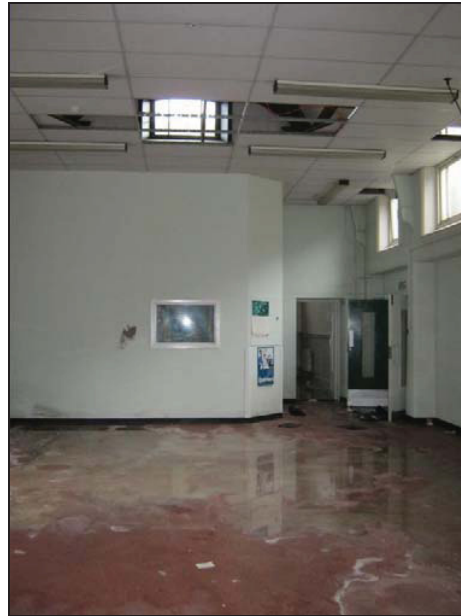
Plate 117 Room 15 Looking Northwest
