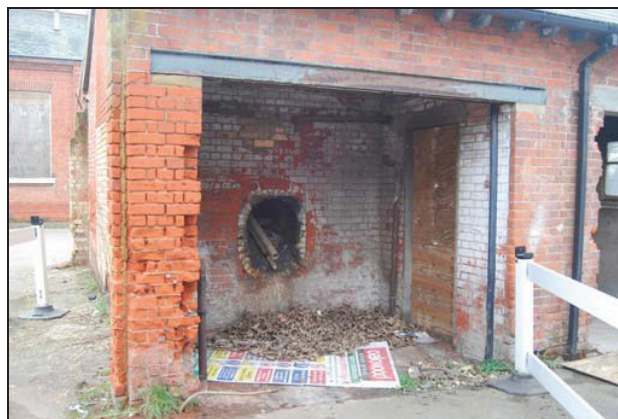
Plate 155: Incinerator area, Looking West
