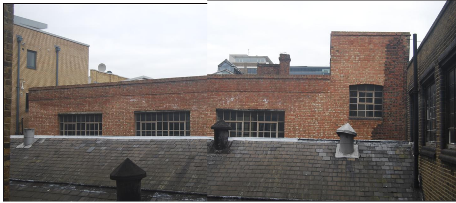
Plate 2: Rear View of Building Showing Repair.
