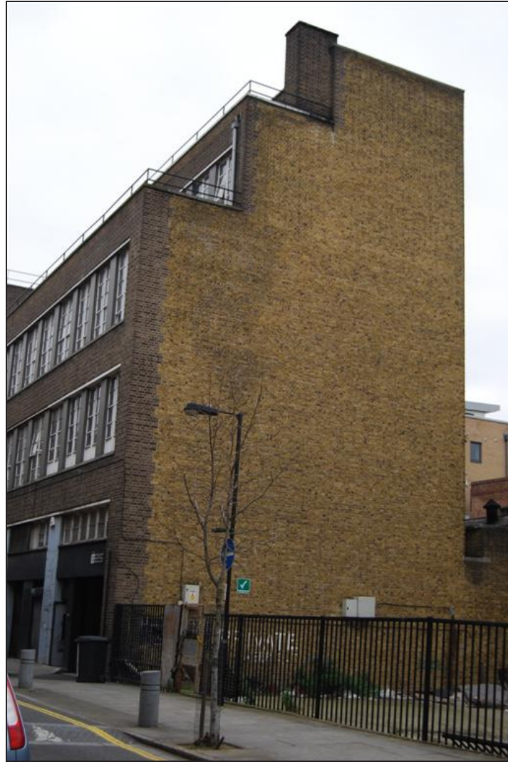
Plate 11: External View of Building on Railway Street, Looking Northwest.
