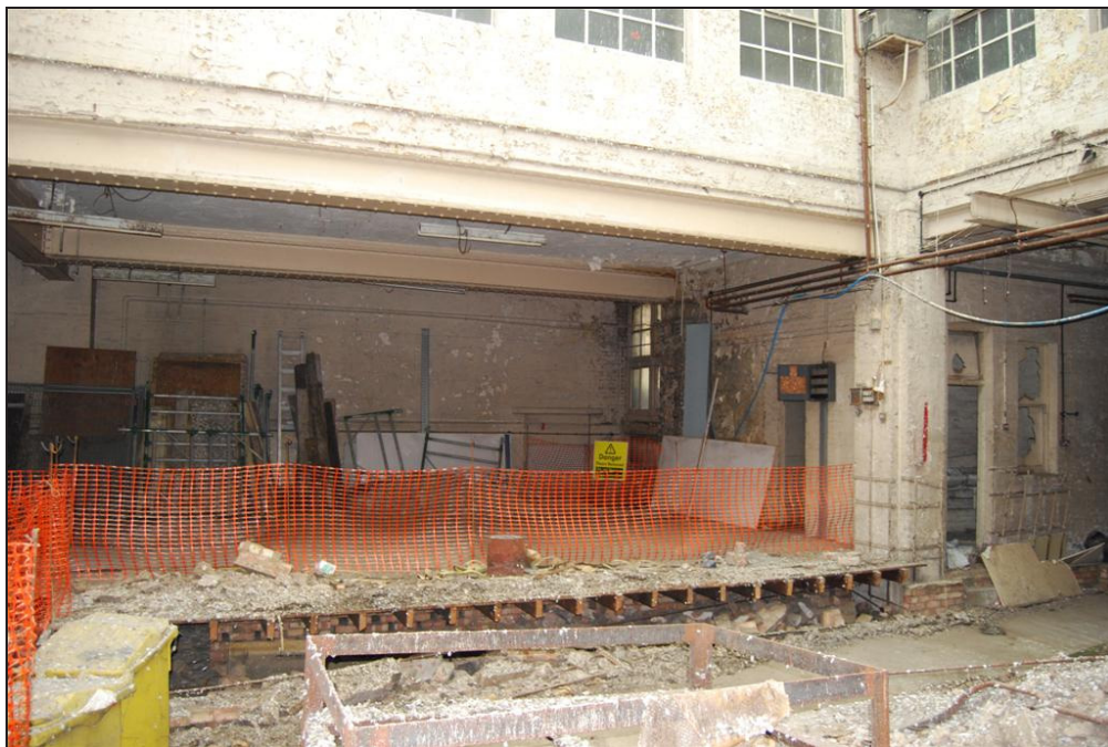
Plate 3: Overview of Warehouse Space, Looking East
