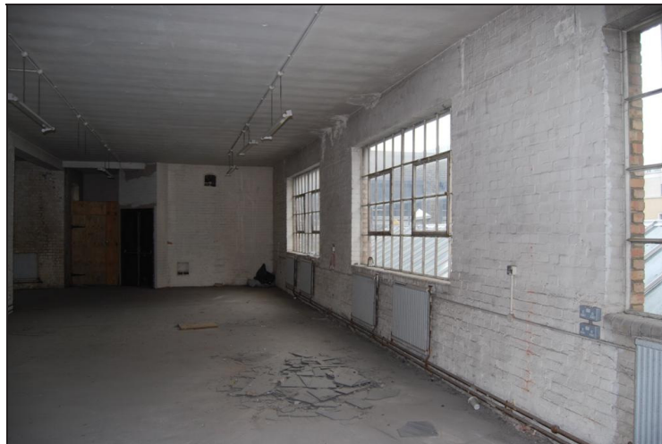
Plate 7: Later Windows in Rebuilt Wall
