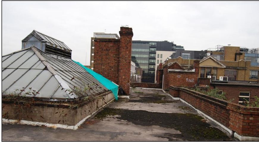
Plate 8: View of Roof Looking North
