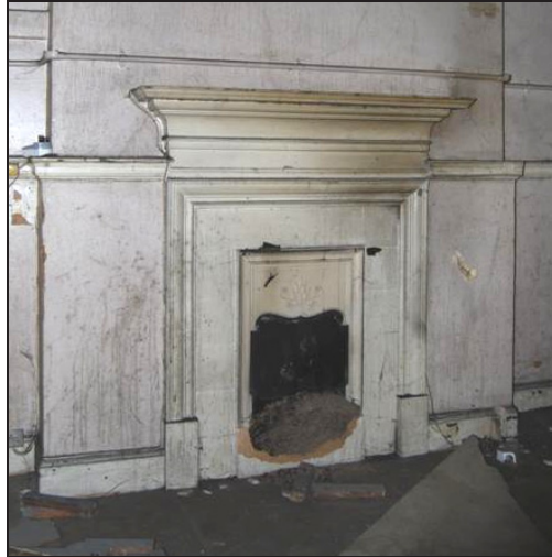
Plate 4: Fireplace in Office
