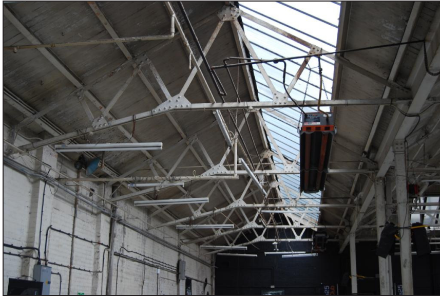
Plate 9: View of Girder Frame, Southern Section Looking West
