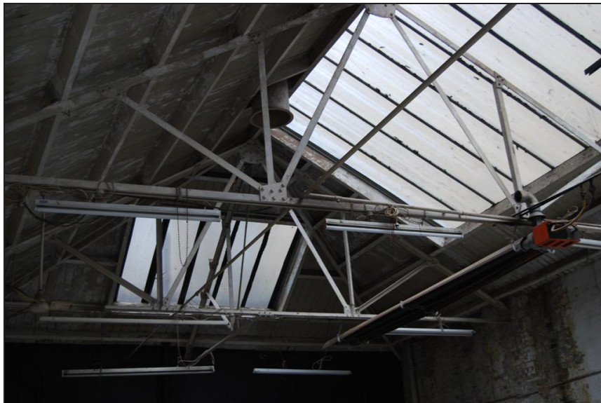
Plate 10: View of Girder Frame, Northern Section, Looking West
