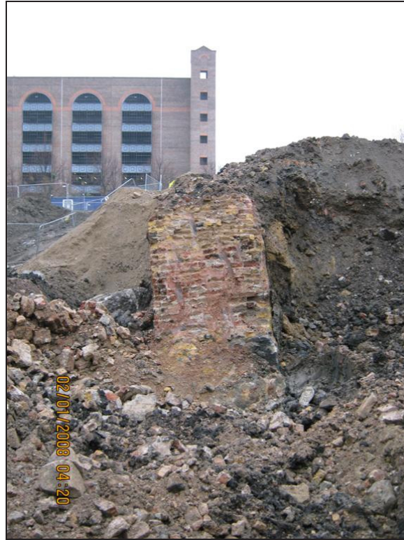
Plate 3: Cut through Dock Wall
