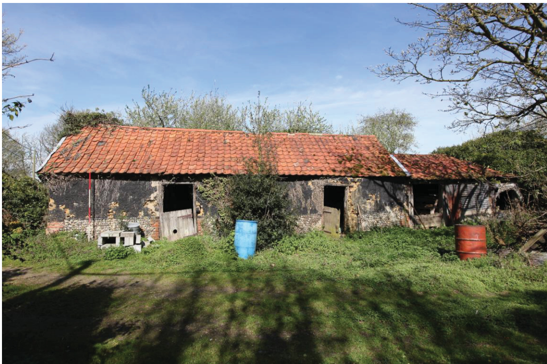
Illus. 2 The southern exterior of the outbuilding showing the clay-lump shed (1) to the left and the boarded shed (2) to the right, both with two entrance doors and pantiled roofs.
