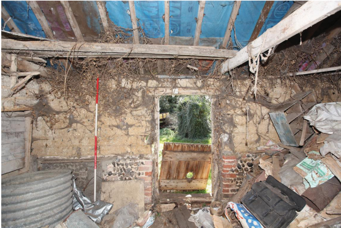
Illus. 5 The southern interior of the western clay-lump shed (1a) showing its original entrance with red-brick dressing to the flint plinth & two bentwood hooks attached to the clay-lump internal partition to the left.
