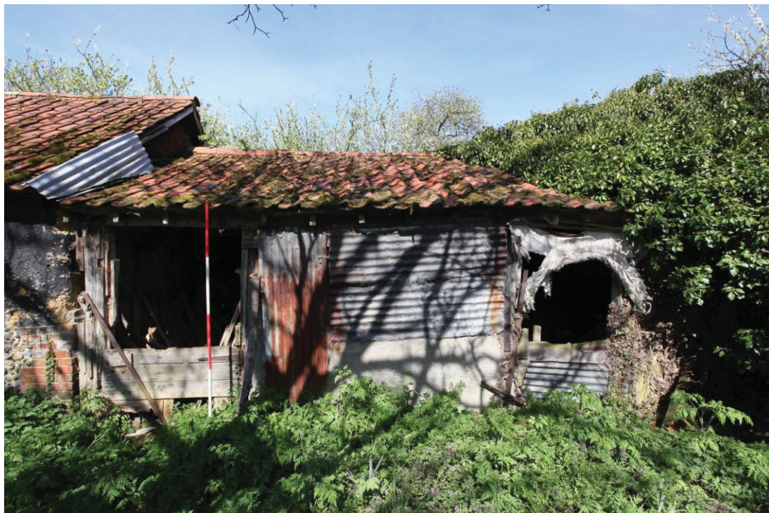
Illus. 4 The southern exterior of the boarded shed (2) showing the 20th century corrugated iron cladding to the western compartment (2a) and the entrance to the eastern compartment (2b) to the right.
