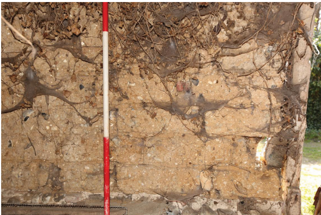
Illus. 6 Detail of the southern interior of the western shed (1a) showing the individual clay-lump blocks laid in clay mortar.
