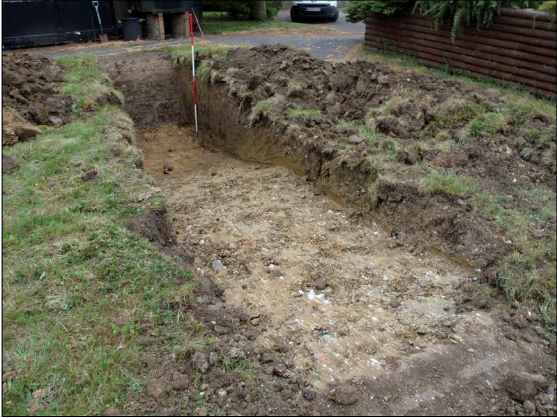
Plate III. Trench 2a, camera facing south west (HGM 99)
