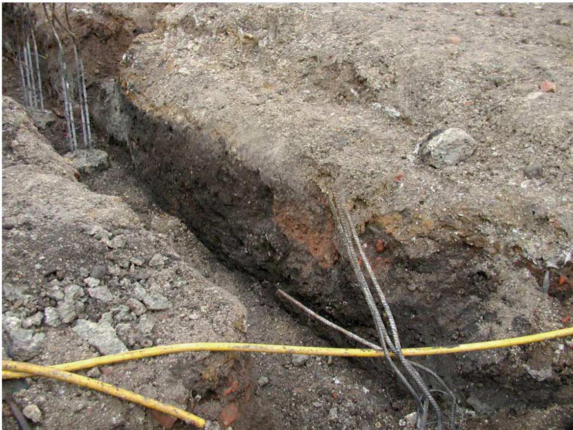
Plate VIII: Sample of ground beam trench (12/4/2005)
