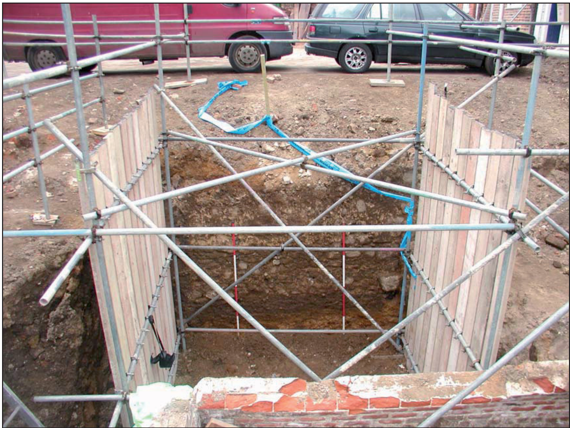
Plate V: Pit excavated for proposed stairwell to cellar (15/3/2005)
