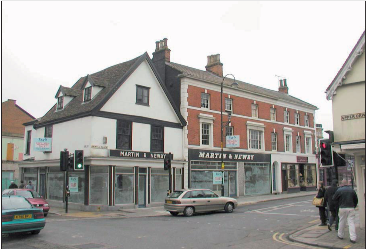
Plate I: General view of the Orwell Place frontage of the former Martin and Newby shop (15/3/2005).
