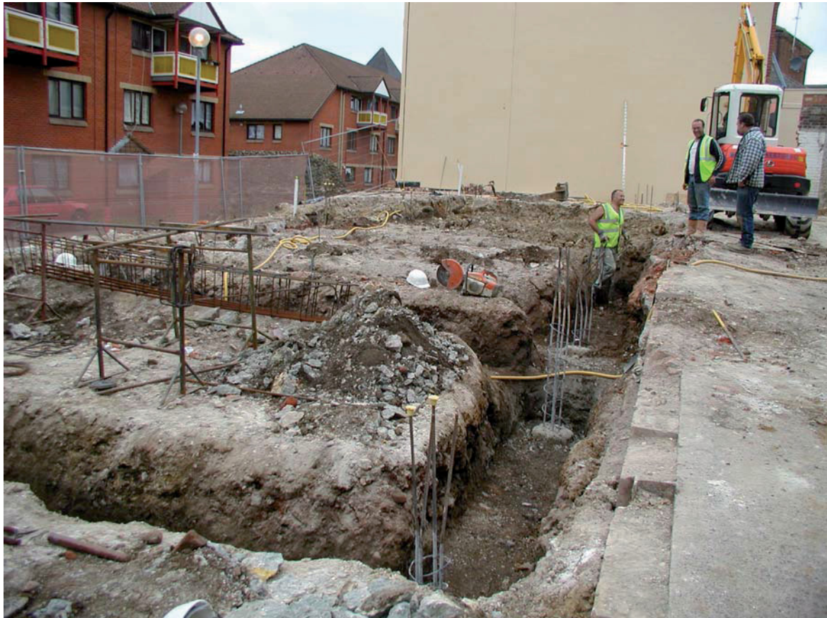
Plate IX: Excavation of ground beam trenches underway (12/4/2005)
