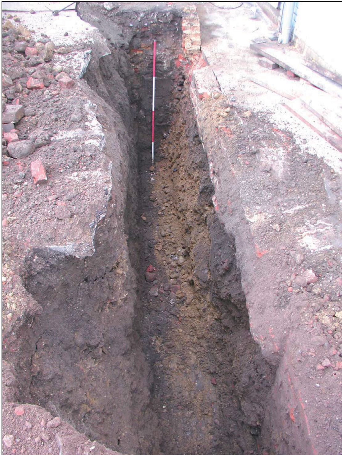
Plate VII: Section of Precinct Wall (0003) revealed in footing trench to the rear of No. 6, Fore Street (10/3/2005)
