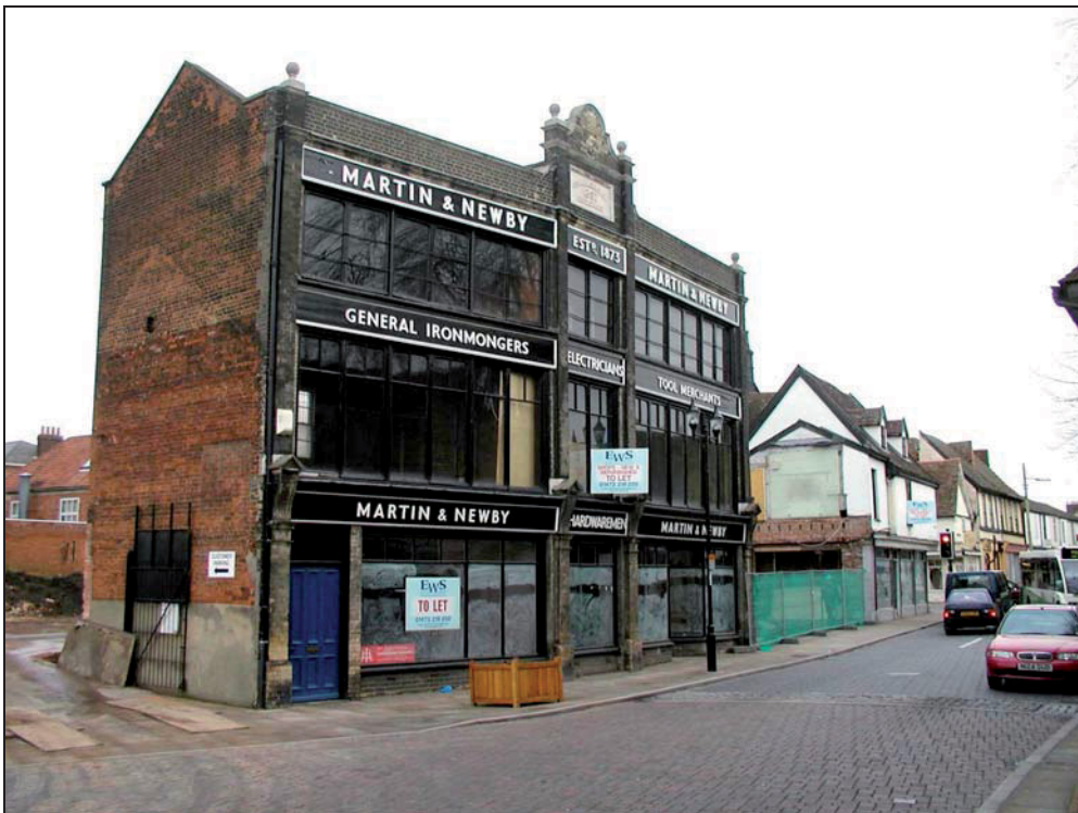
General view of Nos. 4 and 6, Fore Street (11/2/2005).
