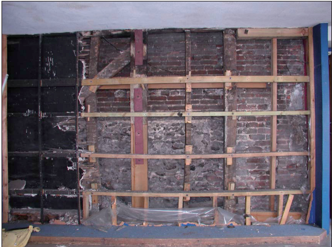
Plate II: Section of Precinct Wall revealed during works within No. 14, Orwell Place (19/8/2004)
