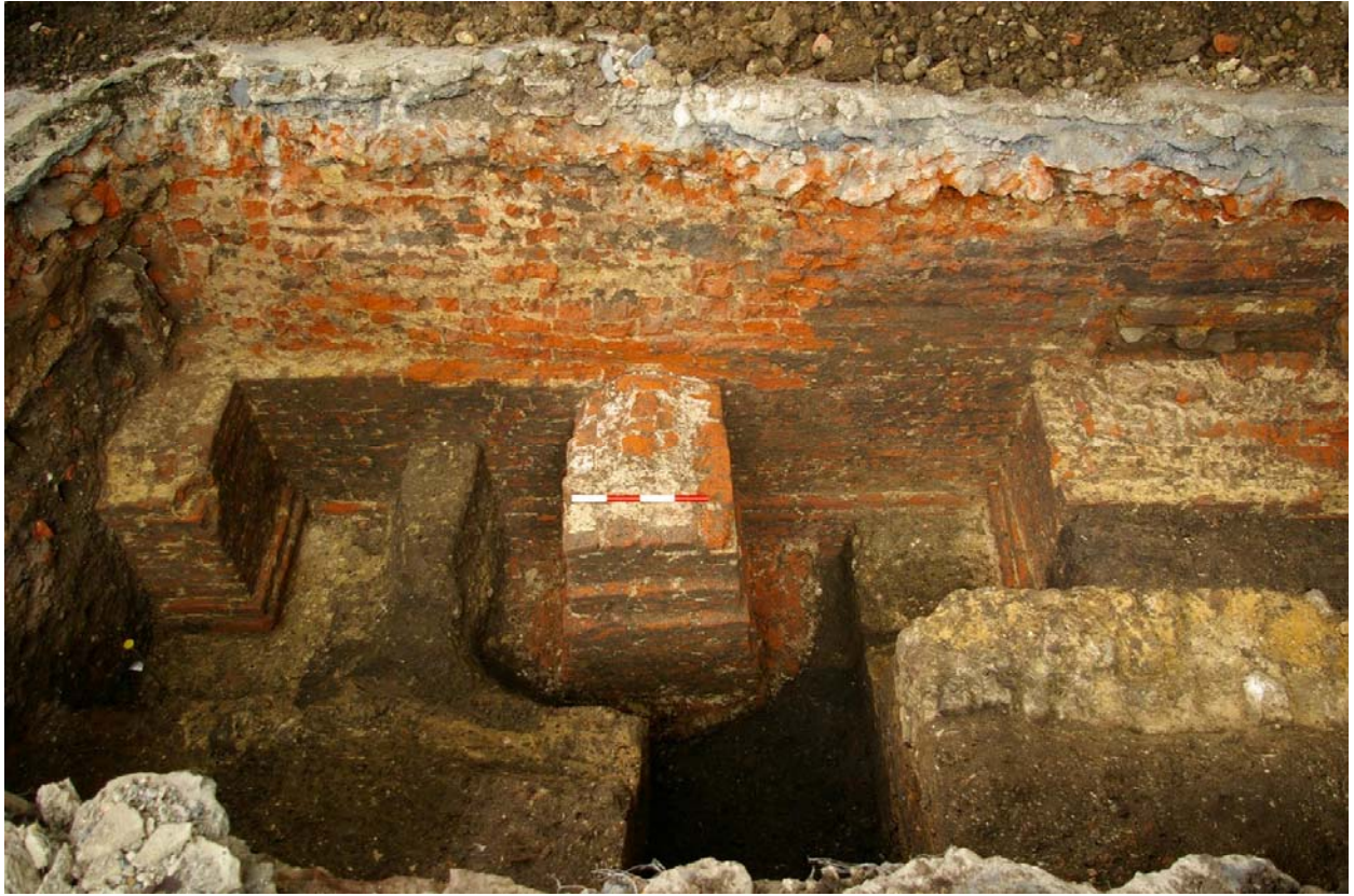
Plate 3. Cellar wall 0146 and associated buttresses (background), and medieval foundation 0189 (right foreground) in Trench 4, looking east (0.4m scale)
