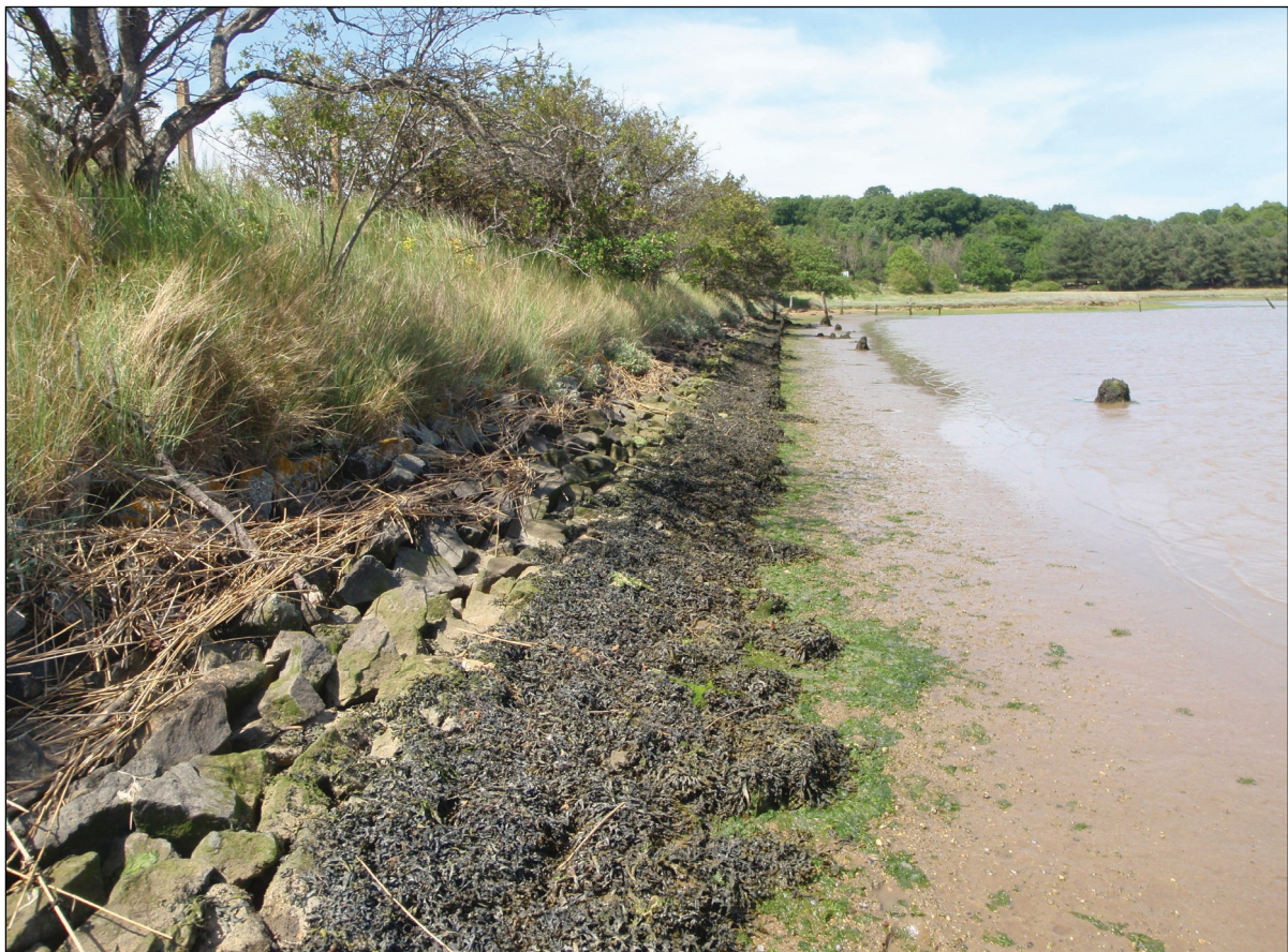
Plate 5. eastern face of the roadside embankment showing the angular stone
