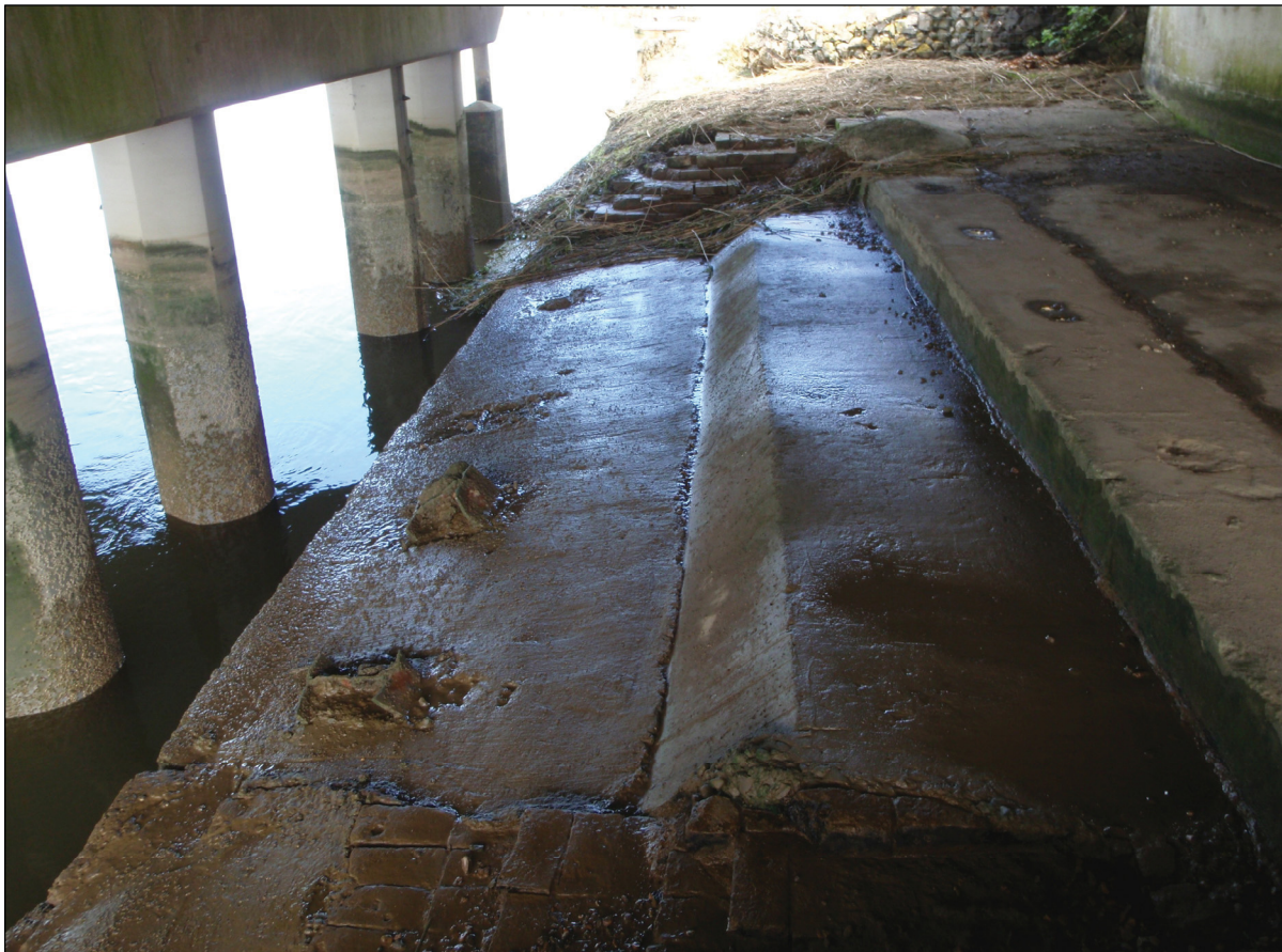
Plate 6. Brick, concrete and girder stumps visible under the south side of the bridge
