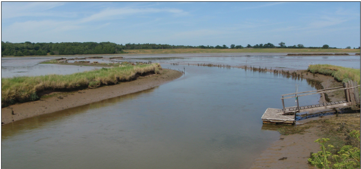
Plate 3. view from Blythburgh Bridge looking east showing the remains of the former river embankments and timber revetments
