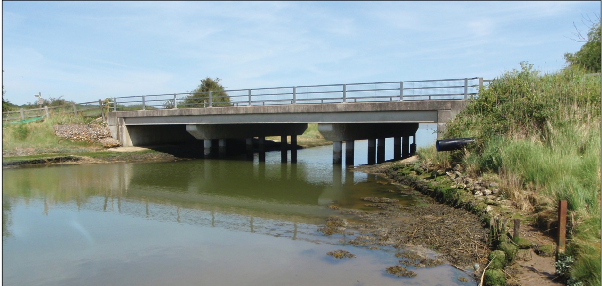
Plate 1. Blythburgh Bridge, west side, looking north-east
