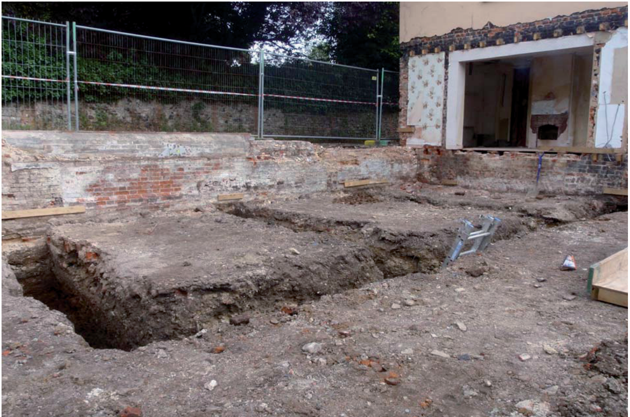
Plate 1. General view of the monitored trenches looking north
