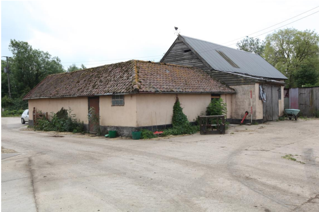
Illus. 3 The farm complex from the north-west showing the 19 th century clay-lump former stable (4) and wood shed (7) in the foreground with the 16 th century timber-framed barn (1) in the rear to right.
