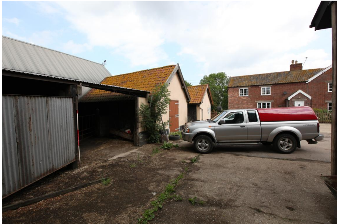
Illus. 5 The eastern exterior of the covered cattle yard (5) from the south-east (left) showing the clay-lump sheds (6 & 7) in the centre and the 18 th century farmhouse with 19 th century brick cladding in the rear to right.
