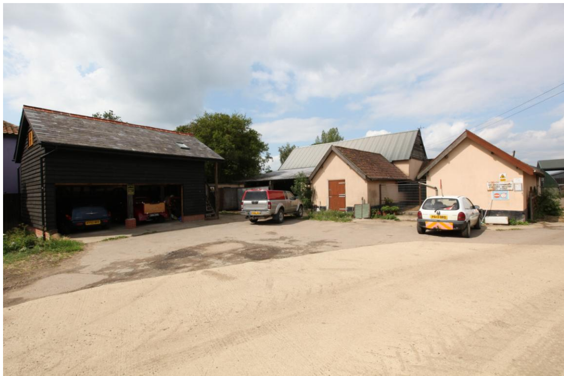
Illus. 2 The Farm complex from the eastern yard flanked by the farmhouse and the previously converted cart lodge and granary shown to the left. The eastern gables of the 19 th century clay-lump shelter shed (6) and wood shed (7), now largely cement-rendered, are visible in the foreground with the 16 th century timber-framed barn (1) in the rear.
