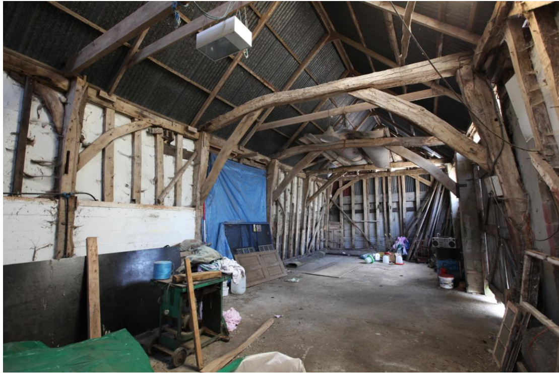
Illus. 7 General view of interior of barn (1) from north showing the largely intact timber frame with original tie-beams and arch-braces but with a 20 th century roof structure. The northern gateway (1a) is shown to the left.
