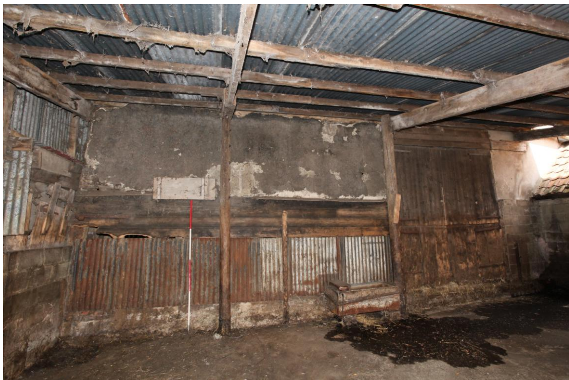
Illus. 6 The eastern exterior of the barn (1) from the covered yard (5) showing its early-19 th century two-tier cladding of tarred lath-and-plaster above weatherboarding and corrugated iron. The 20 th century half-hung doors of the original entrance bay are shown to the right.
