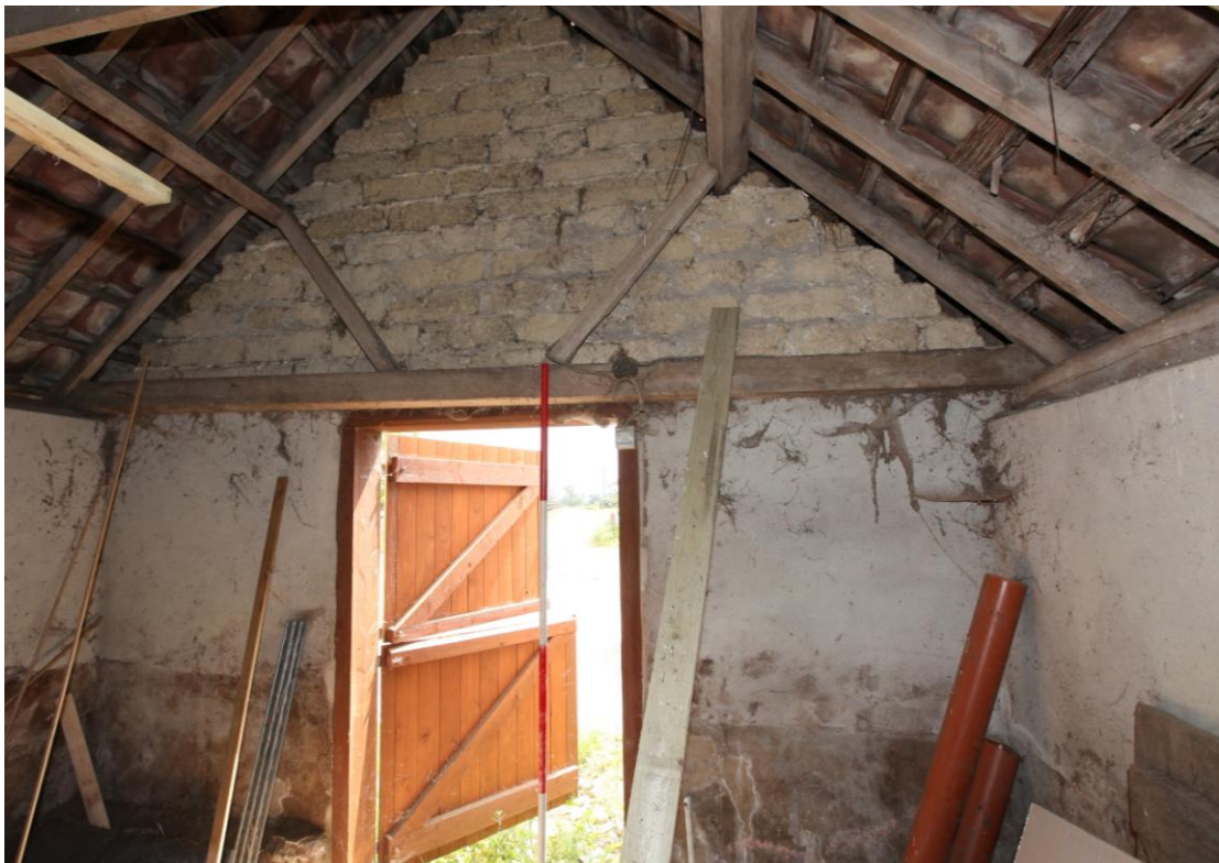
Illus. 4 The internal eastern gable of the clay-lump shelter-shed (6) showing its exposed original clay-lump fabric above the tie-beam and modern door.
