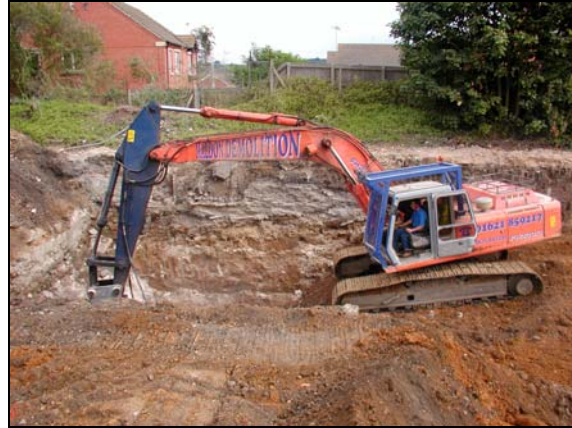
Plate II: final grubbing out of tank (10/8/2005)
