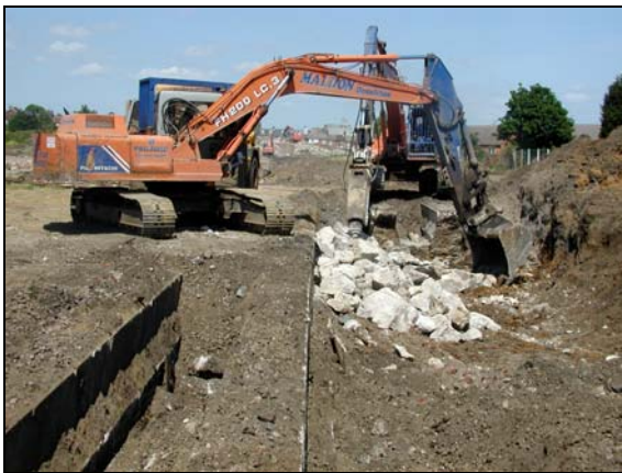
Plate III: Removal of locomotive servicing pits within the former diesel shed (8/6/2005)
