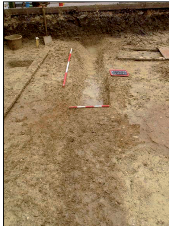
Plate 7. Group 1002 Ditch facing SW (2m & 0.5m scale)
