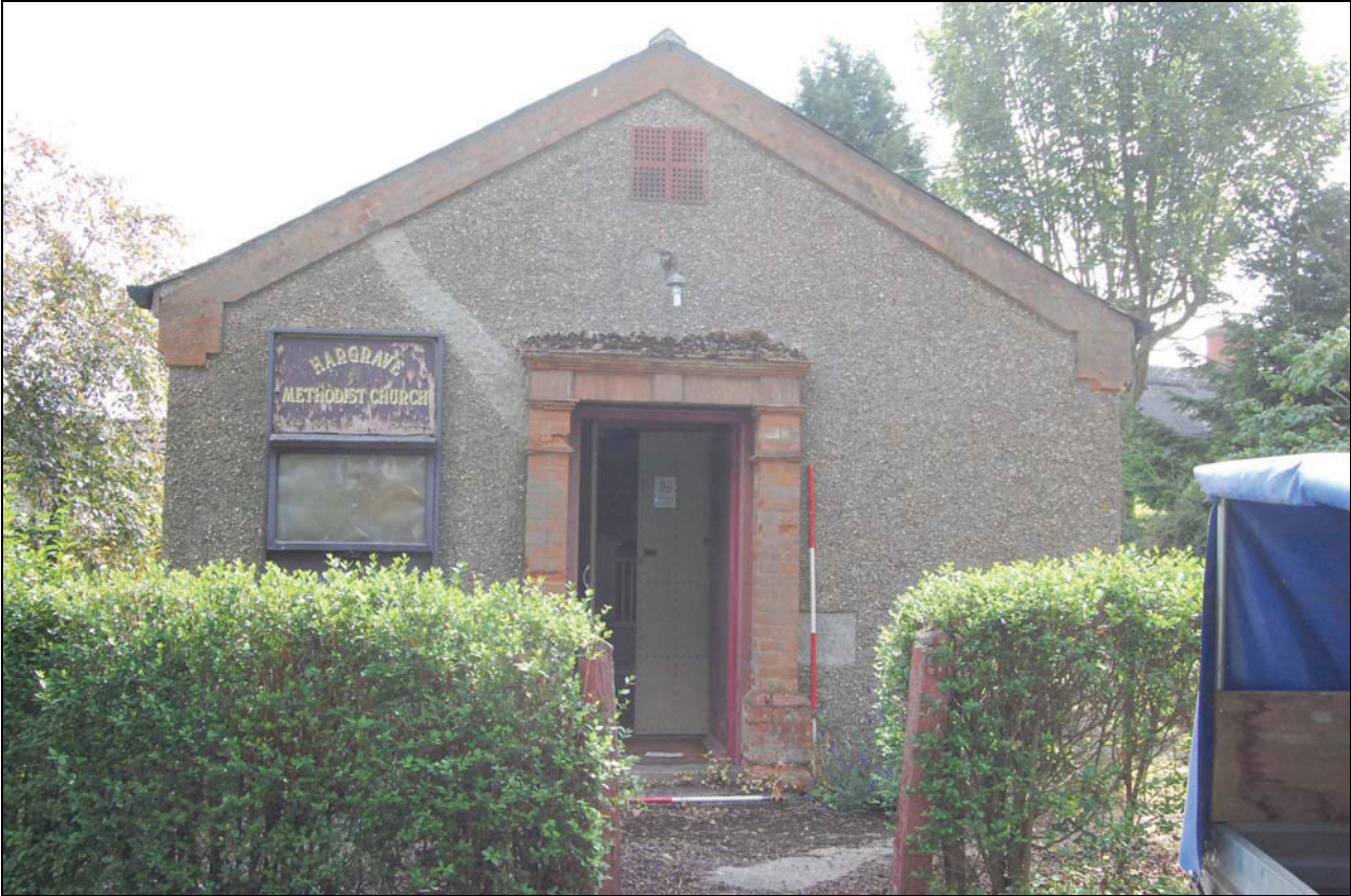
Plate 1. Methodist Chapel, front elevation leading onto Bury Road
