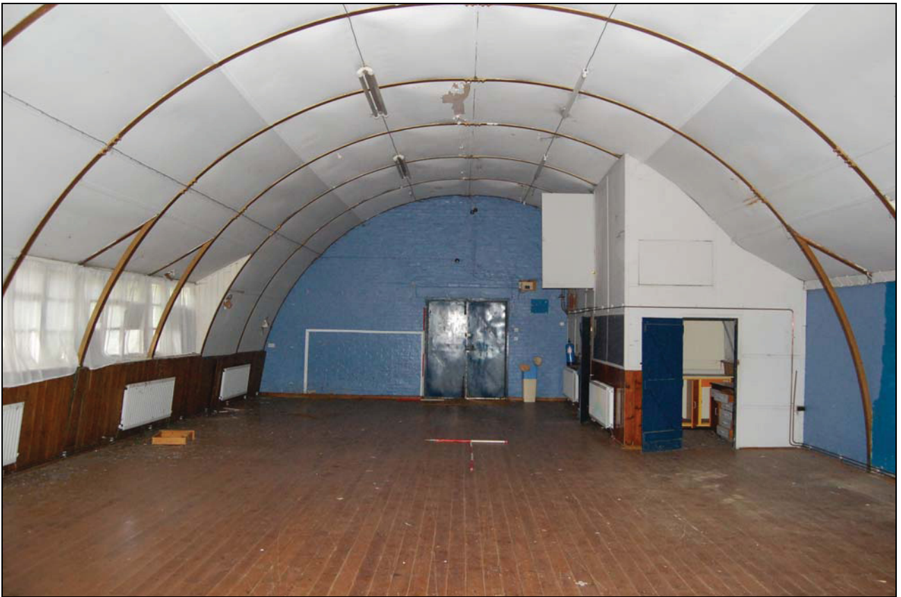
Plate 8. Nissen hut, looking towards entrance and internal rooms, facing WNW
