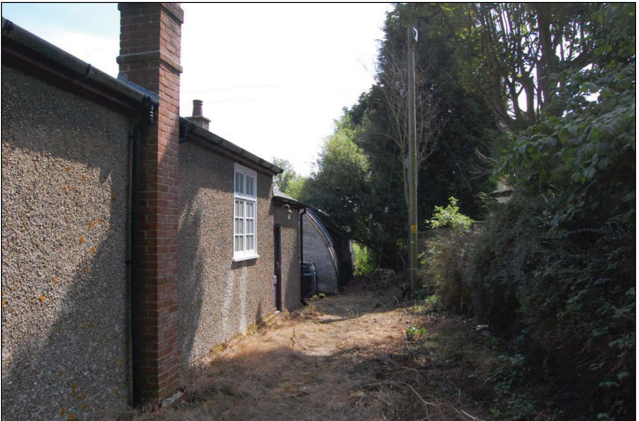
Plate 9. View from Methodist Chapel to Nissen hut, facing E
