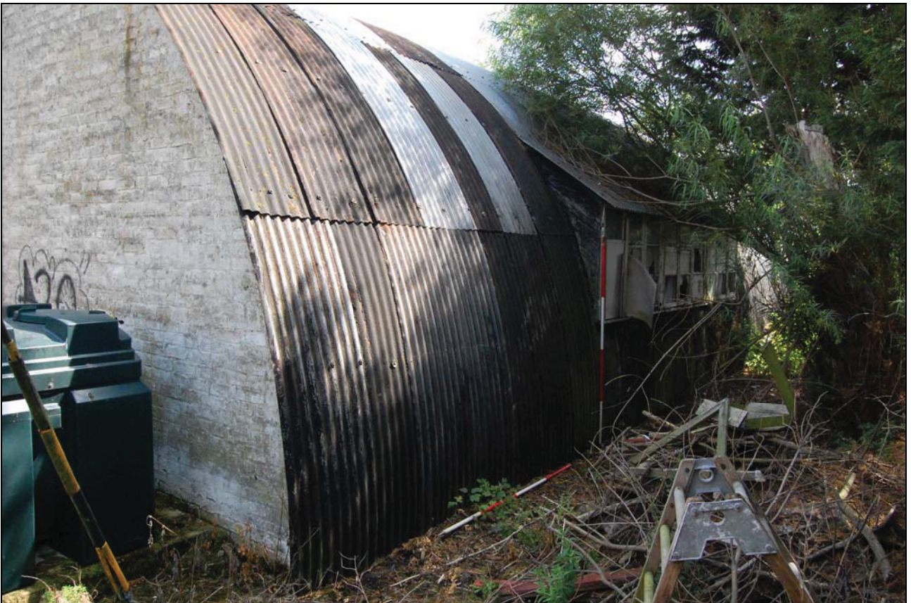
Plate 7. Nissen hut, facing NE
