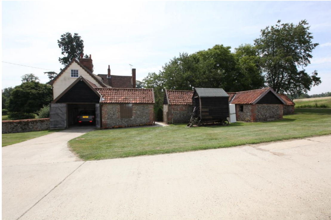
Illus. 3 General view from the north-east showing the single-storied flint-rubble outbuilding (1, 2 and 3) to the right divided by a narrow access (leading to the rear yard and door of the house) from a similar structure with a hinged hatch to the left which lies outside the survey area.
