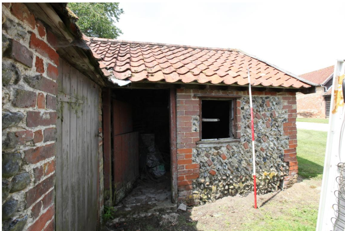
Illus. 6 The eastern exterior of the secondary brew-house (3) showing its original half0hung door and window with the original shed (1) to the left. The letter 'W' is twice boldly incised into the brick dressing to the right of the door.
