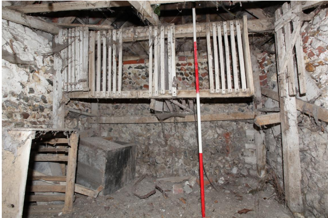
Illus. 11 The good late-19 th or early-20 th century chicken coop of nailed wooden slats with hinged doors attached to the western internal gable of the extension (2b).
