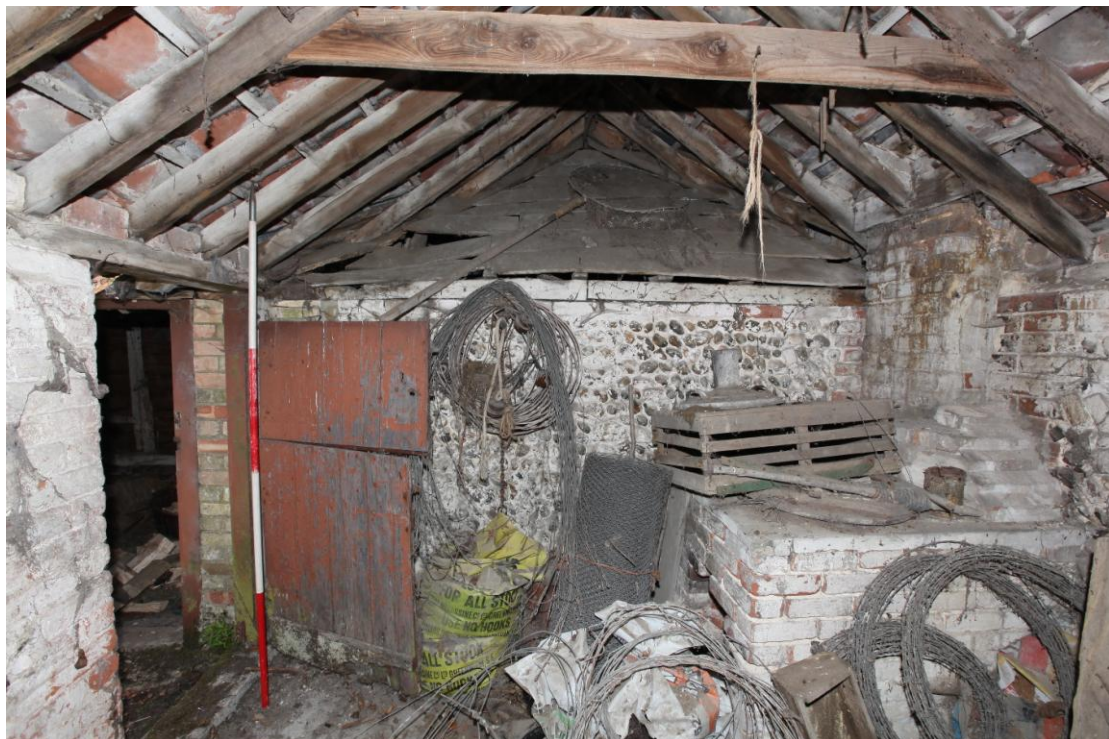
Illus. 12 The southern interior of the brew-house (3) showing the flint-rubble wall of the original shed (1) in the rear with its copper and chimney to the right and half-hung entrance door with red/brown paint to the left. The copper retains its circular boarded lid.
