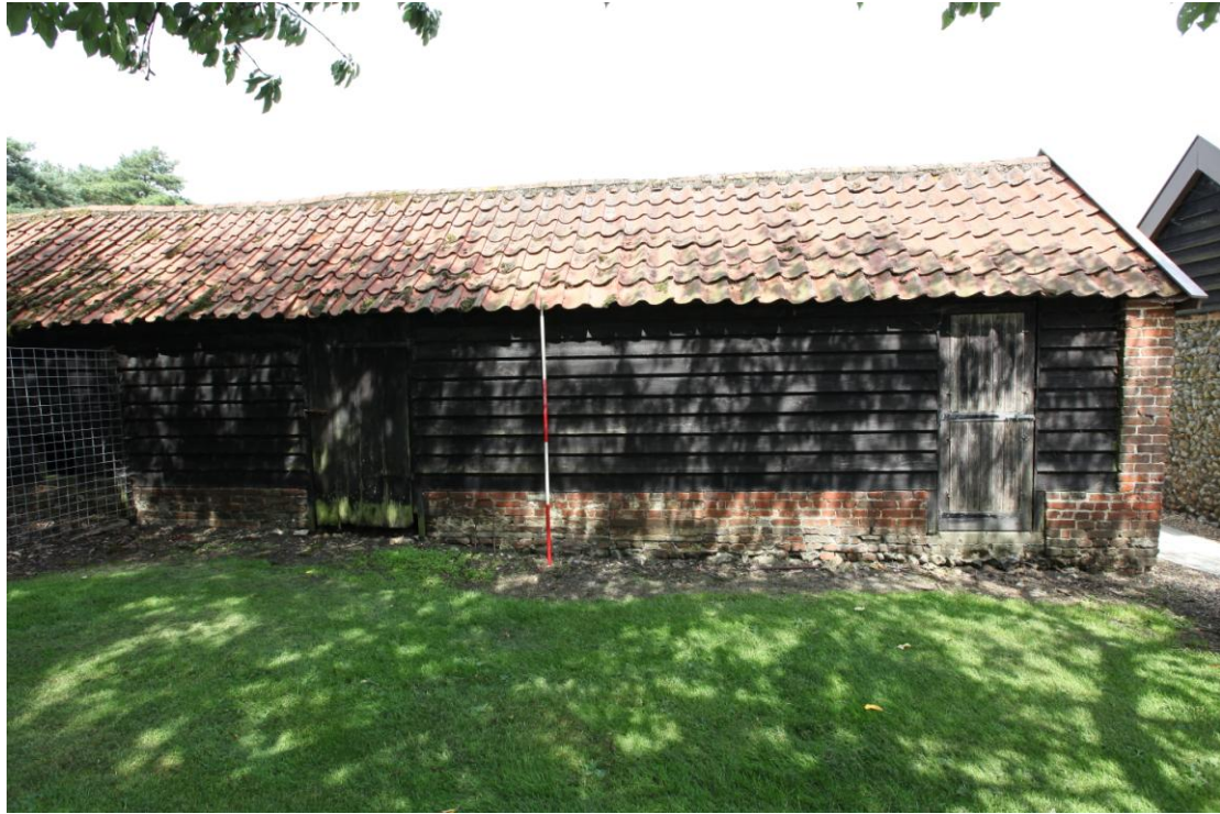
Illus. 7 The weatherboarded southern exterior of the original shed (1) showing evidence of four original entrances.
