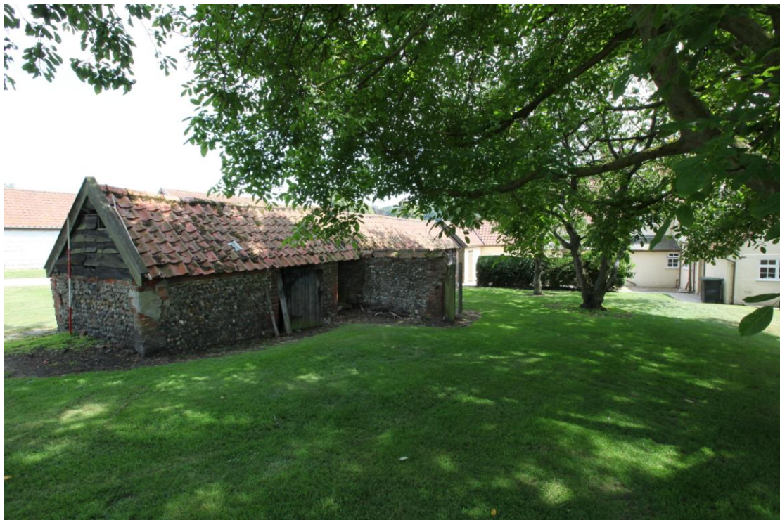
Illus. 4 The exterior from the west showing the later flint-rubble extension (2) to the left with the service yard of the farmhouse in the rear to the right.
