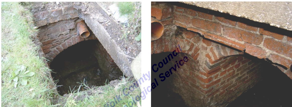
Figure 3. Test pit 2 at junction of culverts
