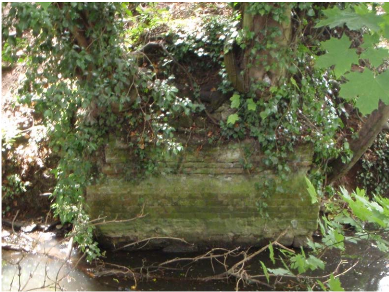
Plate 2. Bridge remains, woodland area, facing west
