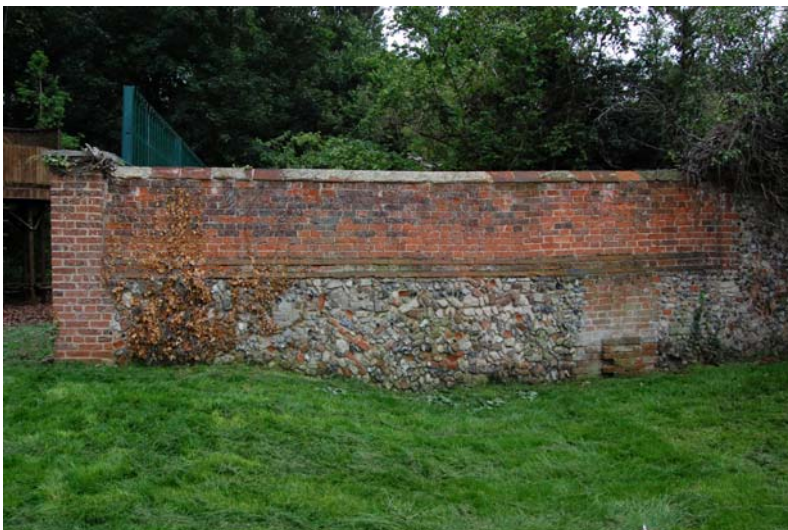
Plate 3. Victorian wall recording, facing south
