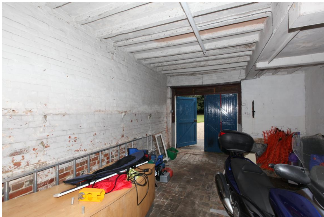
Illus. 8 The interior from the north-east of the central vehicle shed (1c) showing its south-western entrance doors and the lower section of ceiling beneath the domestic bedroom to the right.
