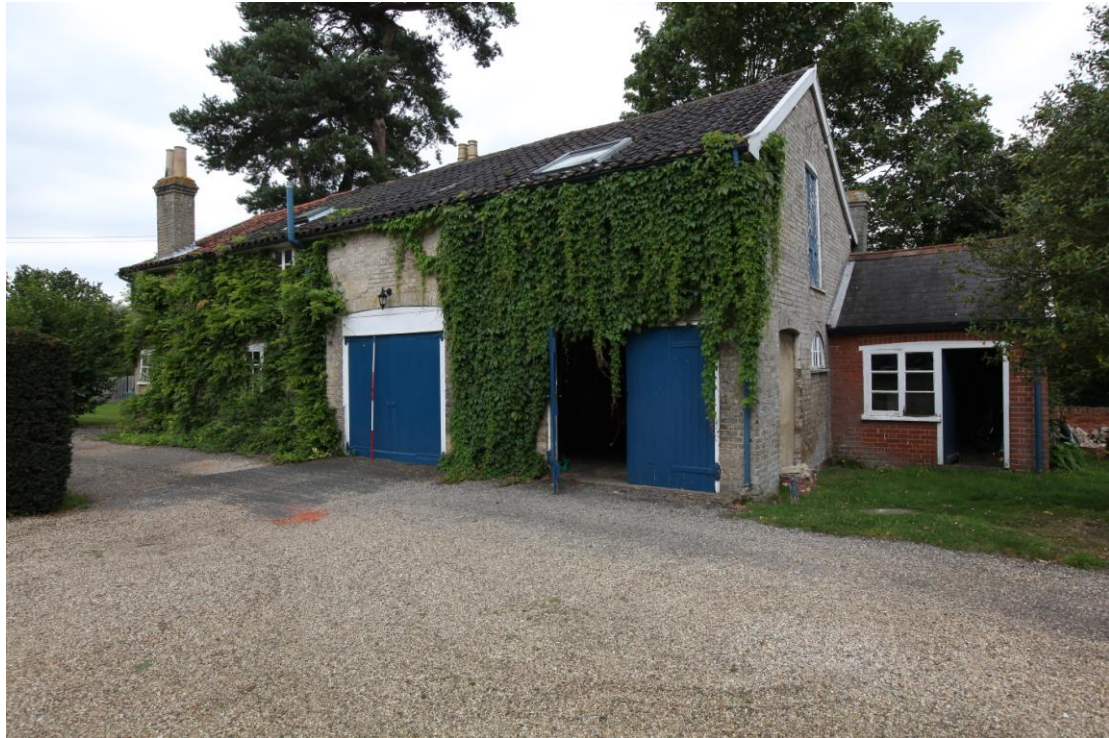
Illus. 3 The south-western facade of Gardeners Cottage showing the doors to the two sheds (1c & 1d) to the right and the domestic cottage windows (1a & 1b) to the left.
