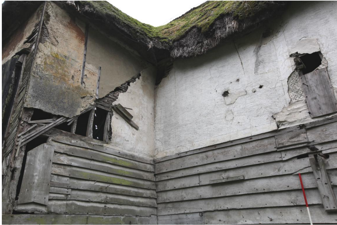
Illus. 3 Detail of the eastern porch (1a) from the west showing the red-ochre pigment above the scar of the demolished lean-to (left) and the herringbone pargeting to the original unpainted lime plaster of the barn to the right. The absence of pargeting beneath the scar on the porch indicates the porch and lean-to were contemporary additions to the earlier barn.
