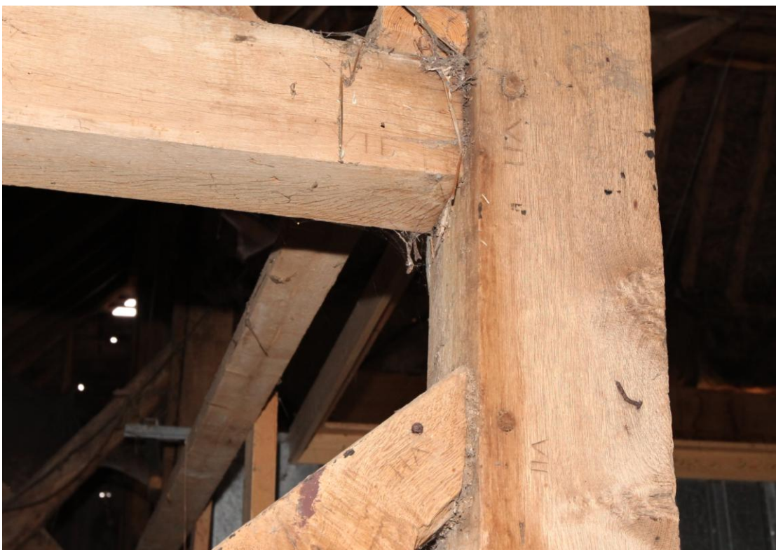
Illus. 10 A detail from the east of the lateral truss to the west of bay H (as in illus 9 above) showing the identical chiselled Roman carpenter's numerals (VII) to all original components. The northern storey post of the truss bears the same number.
