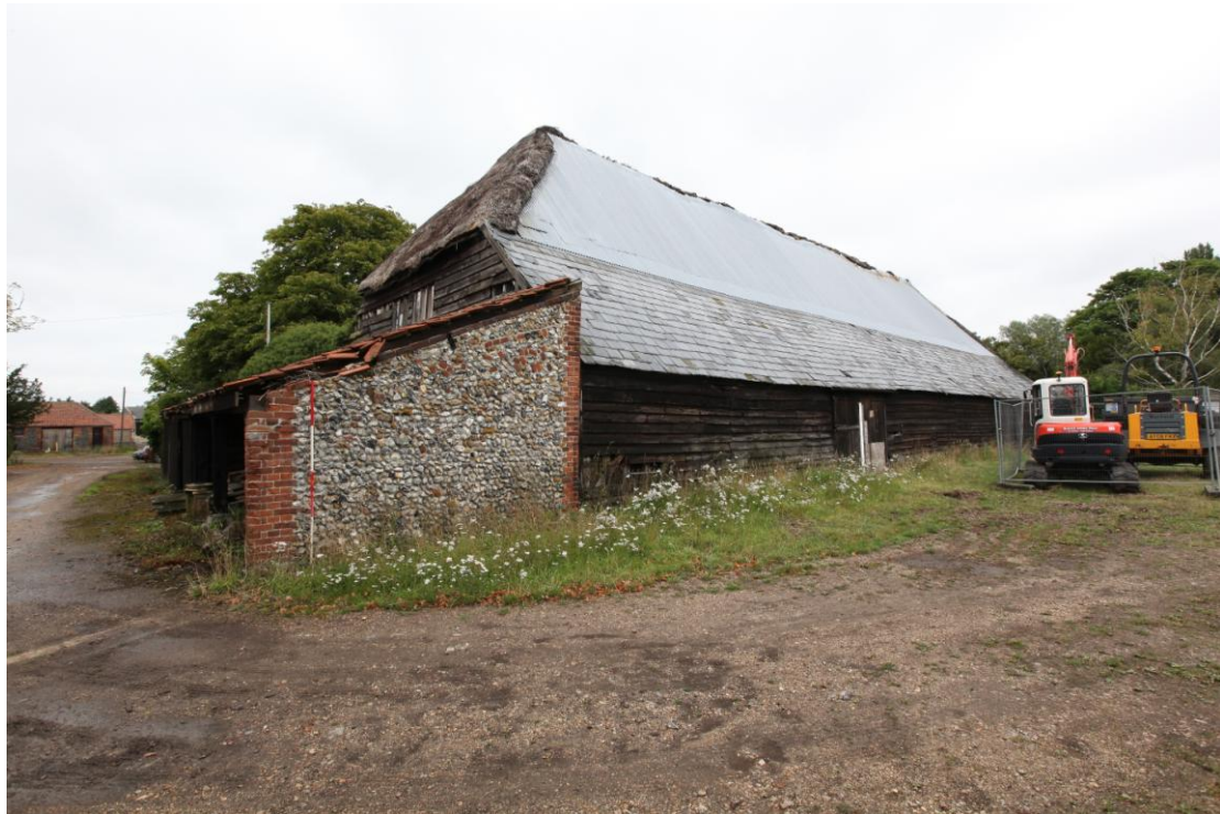
Illus. 4 The exterior of the barn from the south-west showing the flint-rubble lean-to (3) to the left and the slate roof of the rear (southern) aisle beneath the modern corrugated metal which has replaced the thatch to this elevation.
