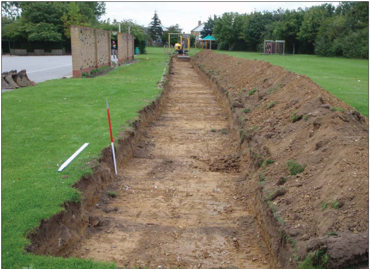
Plate 1. View of Trench 1, looking west.
