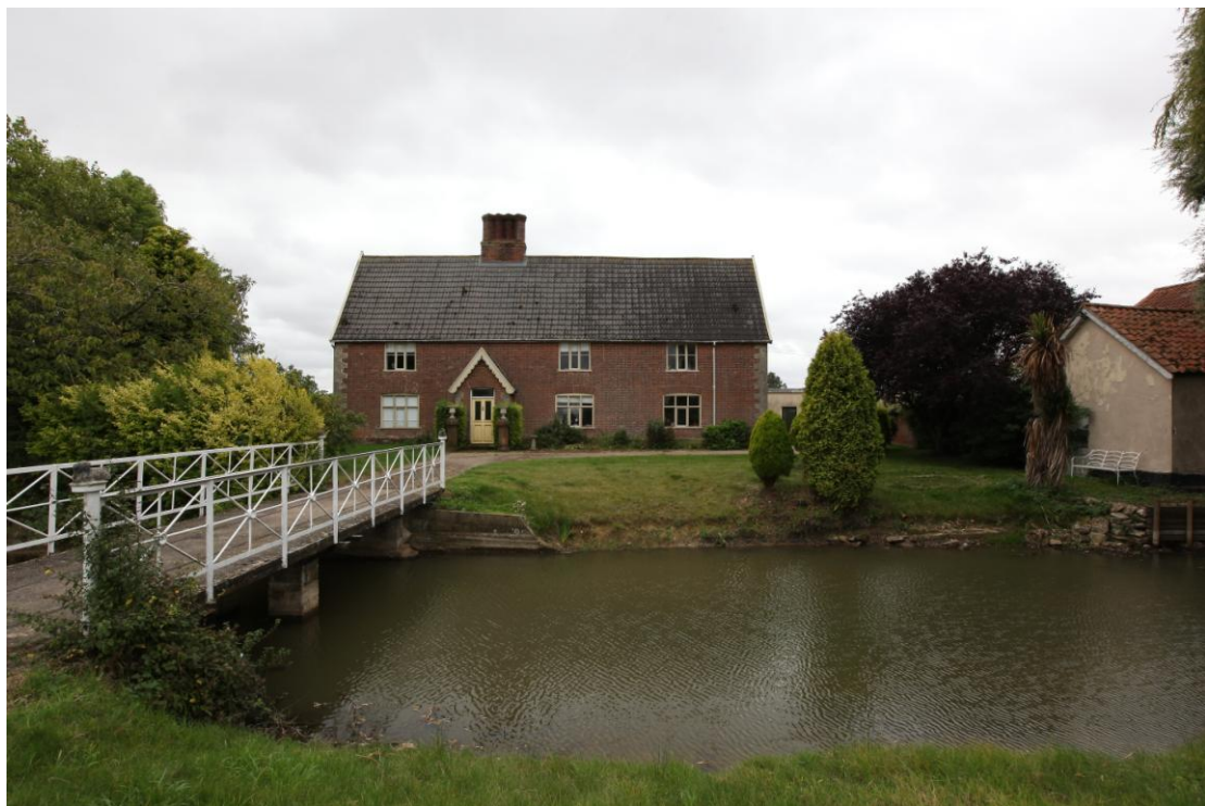
Illus. 2. The grade II-listed farmhouse of circa 1600 with its 19th century brick facade seen from across the moat to the north. Included for site context.
