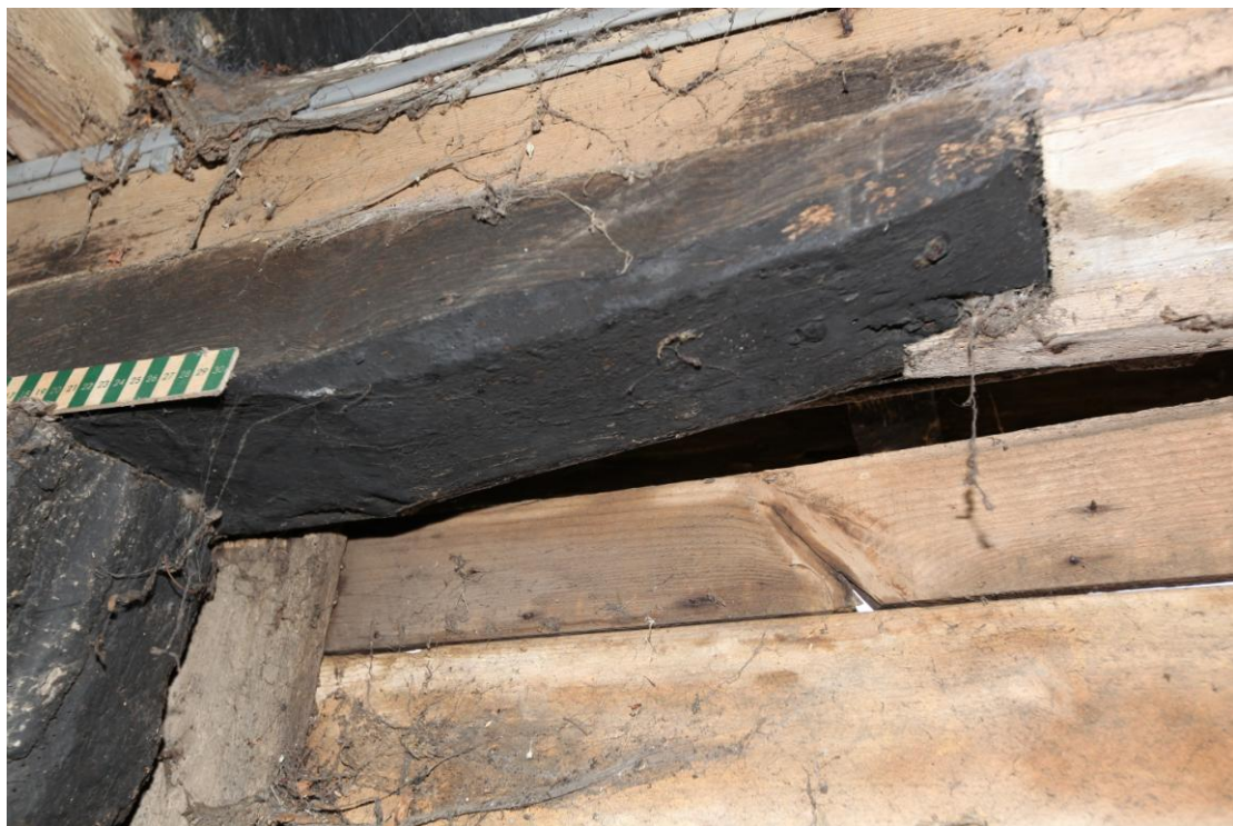
Illus. 10. Detail of the northern chamfered arcade post lintel of the eastern interior showing the heads of the iron nails which secure it to the roof-plate.
