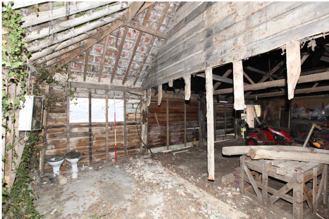
Illus. 6. The northern bay from the west showing the narrow inserted studs without a brace to the formerly open eastern elevation, and the remains of the original internal partition to the right.
