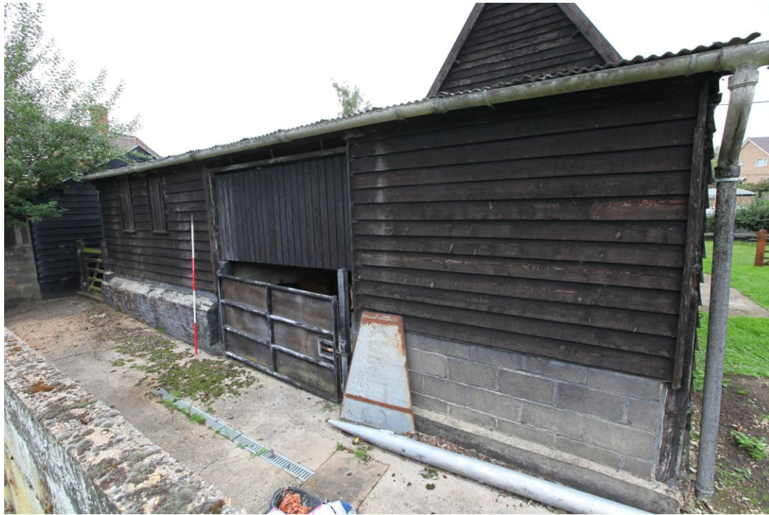
Illus. 5 The eastern exterior which was almost entirely rebuilt in the late-20th century to incorporate what appears to be an entrance gate for cattle with glazed windows to the southern shed (F) to the left.
