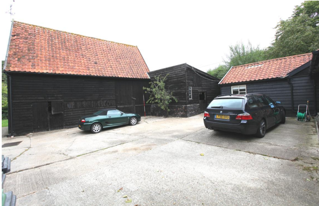
Illus. 3 General view of the site from the concrete yard to the south-west showing the doors to the floored bays (A & B) to the left and the barn doors to the right. The roof of the southern shed (F) in the centre was originally of the same pitch and height as that of the barn but has been truncated.
