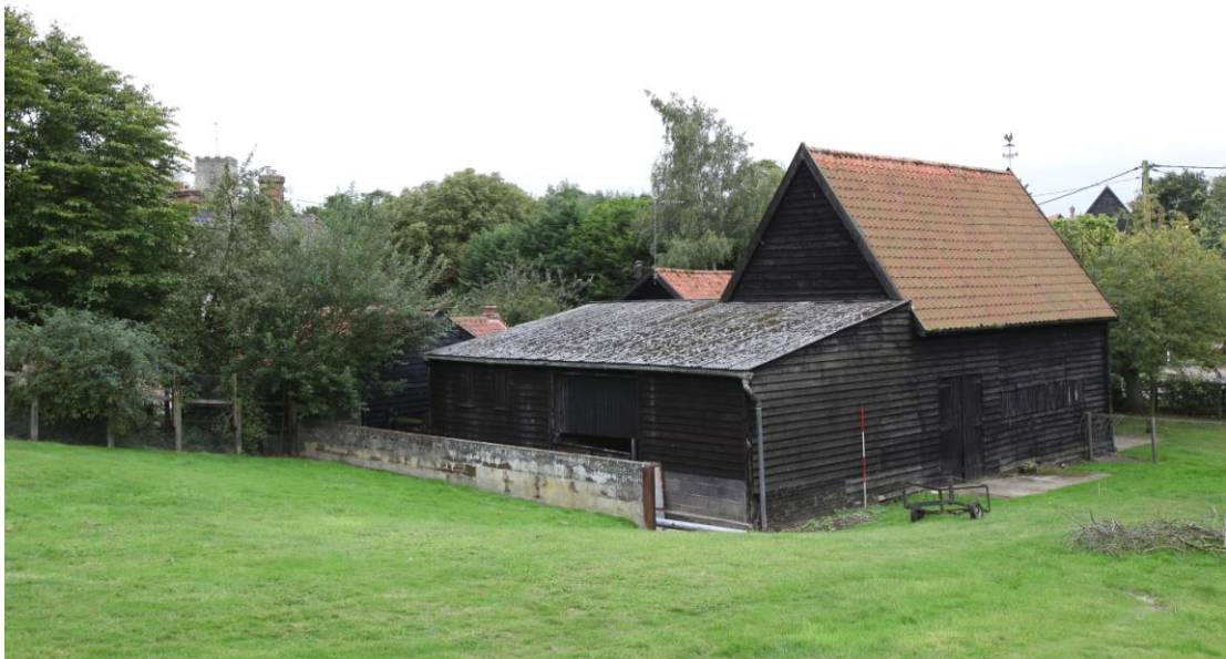
Illus. 1 General view of the site from the north-east showing the church tower to the left and the gable of Church Farm Stables in the rear to the right. The steeply pitched pantiled roof of the barn was originally thatched and extended further to the left but was truncated in the 20 th century to form the present ‘lean-to’.
