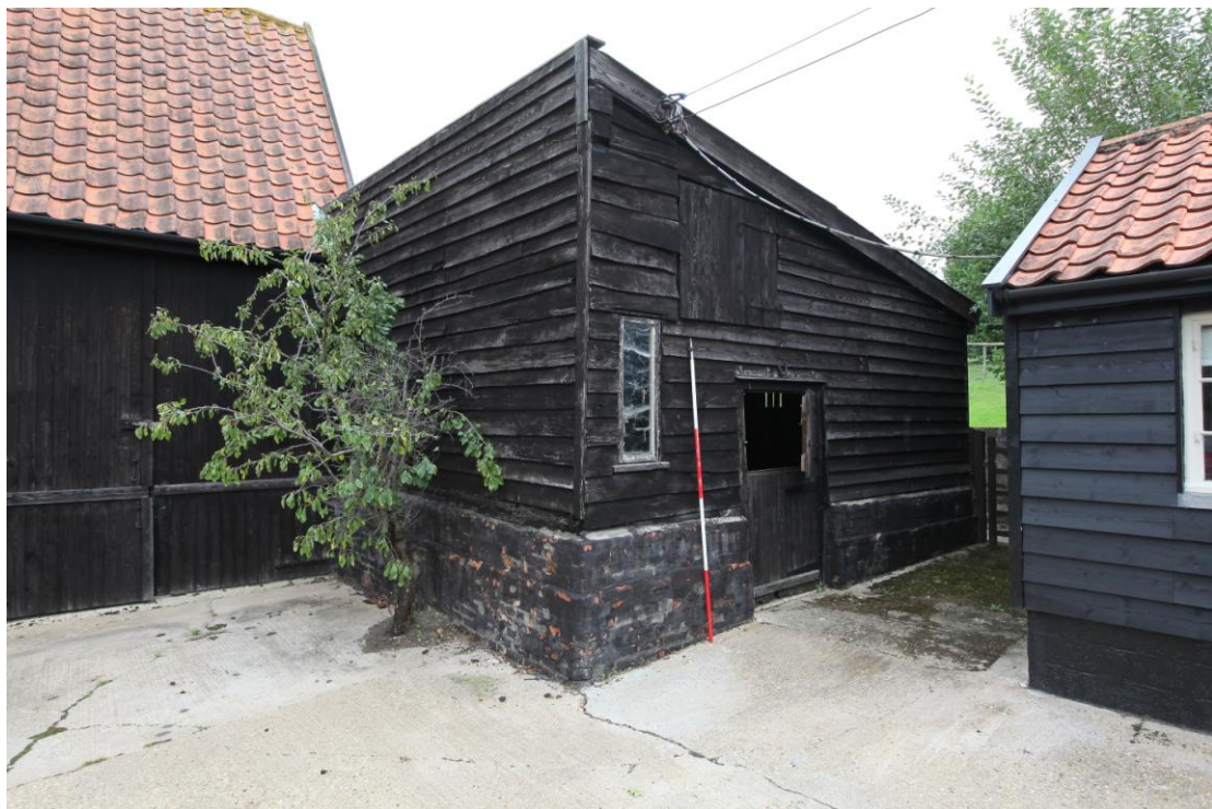
Illus. 6 The exterior of southern shed (F) from the south-west showing its truncated roof and the loading hatch to the loft. This gable was originally of identical proportions to the western gable of the barn and the apexes of the two roof structures would have met at right-angles.
