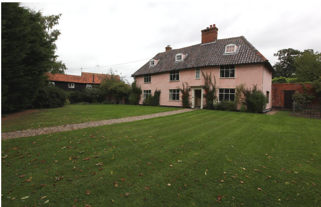
Illus. 2 General view of the site from the south-west showing the high roof of the barn to the left of Willow House (a grade II-listed timber-framed and rendered structure of circa 1640 with a central hall flanked by a parlour to the right and a service bay to the left).
