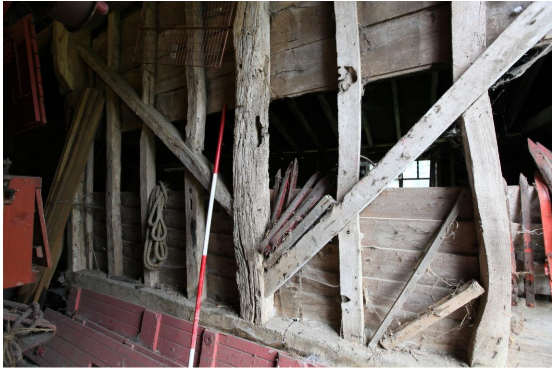
Illus. 9 The northern interior of the eastern bays of the barn (1) showing a typical section of wall fabric: The diagonal primary braces which interrupt the vertical studs are tenoned and pegged to the intermediate post in the centre. Many timbers, including the weathered post, contain empty mortises and have been re-used from earlier buildings.
