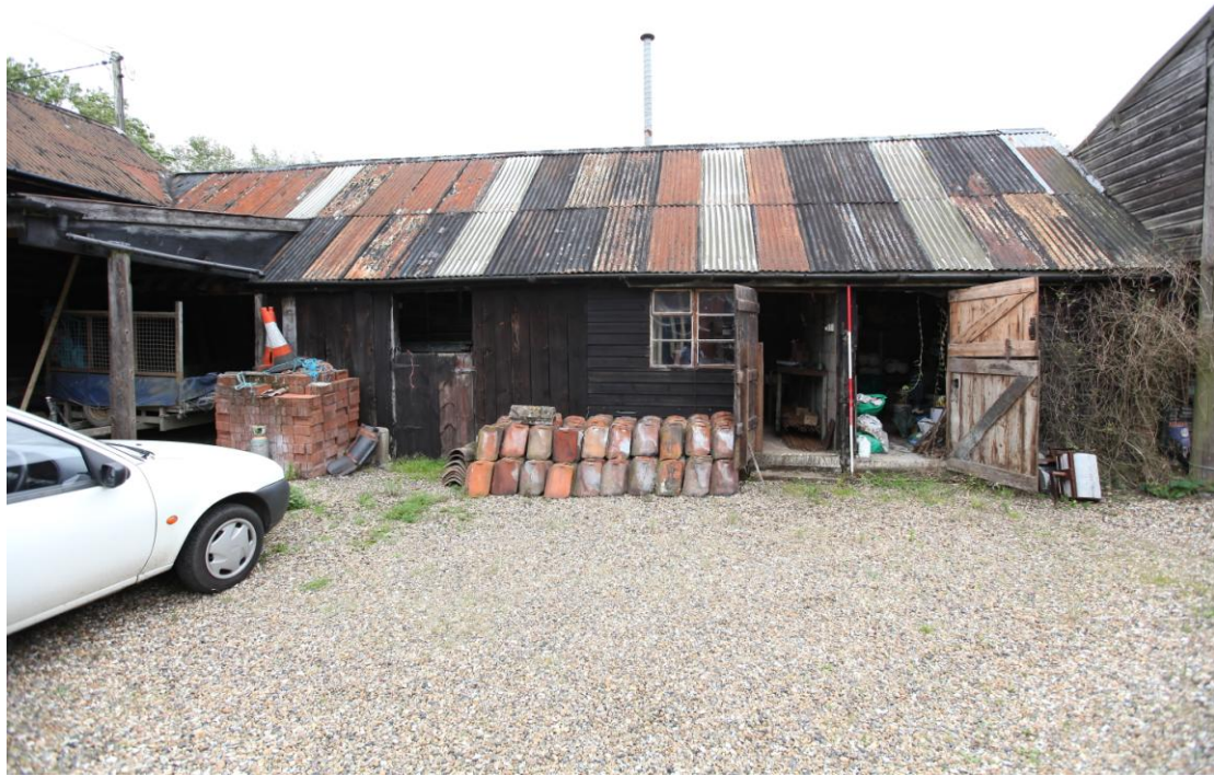
Illus. 5 The originally open western exterior of the brick shelter-shed (4) showing its 20th century boarded infill and corrugated iron roof.
