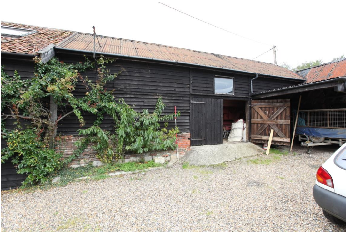
Illus. 4 The southern exterior of the barn (1) showing its 20th century weatherboarding and central doors with the original brick plinth contained re-used ashlar (dressed stone) to the left.
