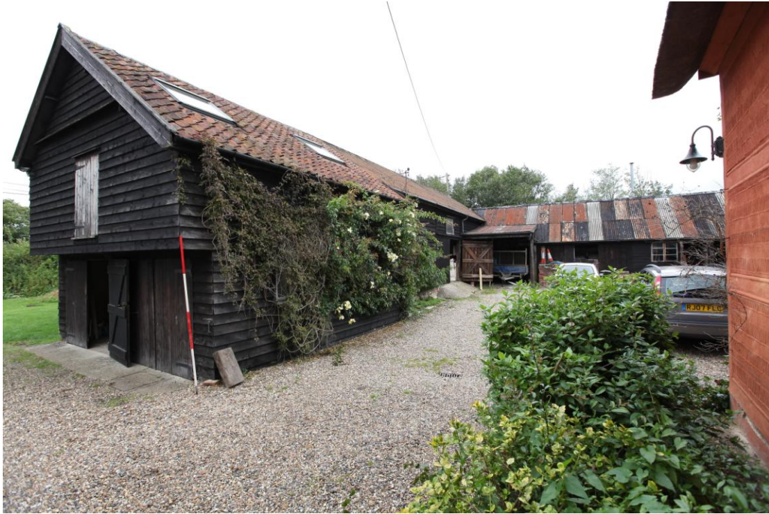
Illus. 3 The exterior from the west showing the unlisted but reputed 17 th century farmhouse to the right with the brick shelter-shed (4) in the centre and the barn (1) and 1980s garage (2) to the left.
