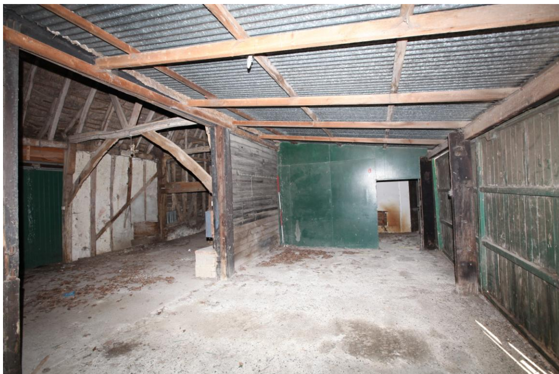
Illus. 4. The interior from the west of the 20th century lean-to shed (2) showing one of its two internal partitions and the tarred and weatherboarded southern exterior of the barn (1) to the left. The storey posts of the entrance in the central bay (1a) bear iron pintles for missing half-hung barn doors.
