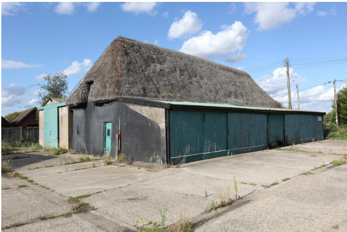
Illus. 2. The exterior from the south-west showing the fully hipped and thatched roof of the barn (1) in the centre with the late-20 th century lean-to with sliding doors (2) to the right and the garage shed (3) to the left.
