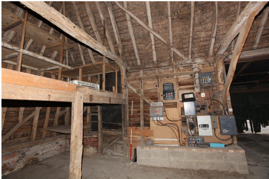
Illus. 10. The southern interior of the slightly later eastern bay of the barn (1b) showing its rebuilt loft with black-painted loading hatch and half-hung entrance door in the centre. The adjoining tie-beam of the threshing barn contains empty mortises for the studs of its missing eastern gable.
