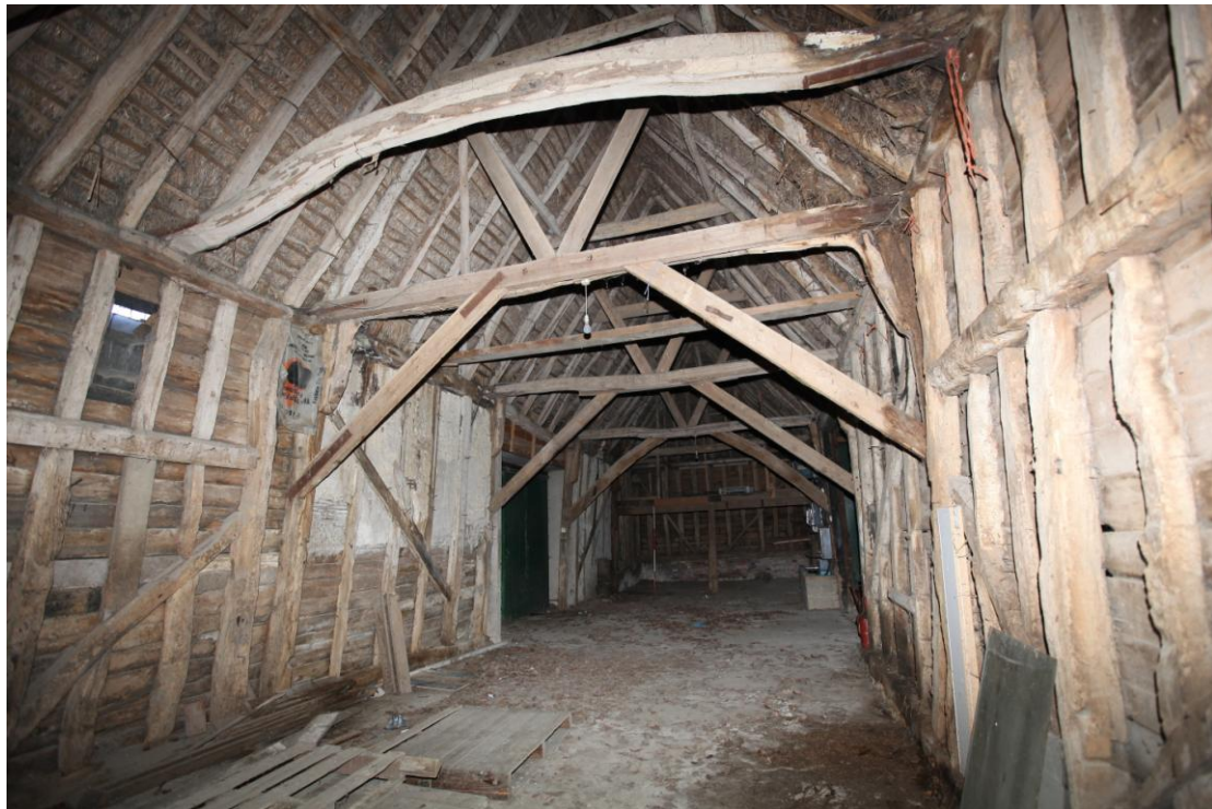
Illus. 6. General view of the barn interior from the west showing two secondary pairs of arch-braces to the tie-beams in the foreground and an original pair in the rear. The interior was originally divided into three compartments by lateral partitions that have since been removed, viz. a three-bay stable and hay loft in the foreground (1c), a slightly earlier three-bay threshing barn in the centre (1a) and a narrow floored bay that may have served an additional stable in the rear (1b).
