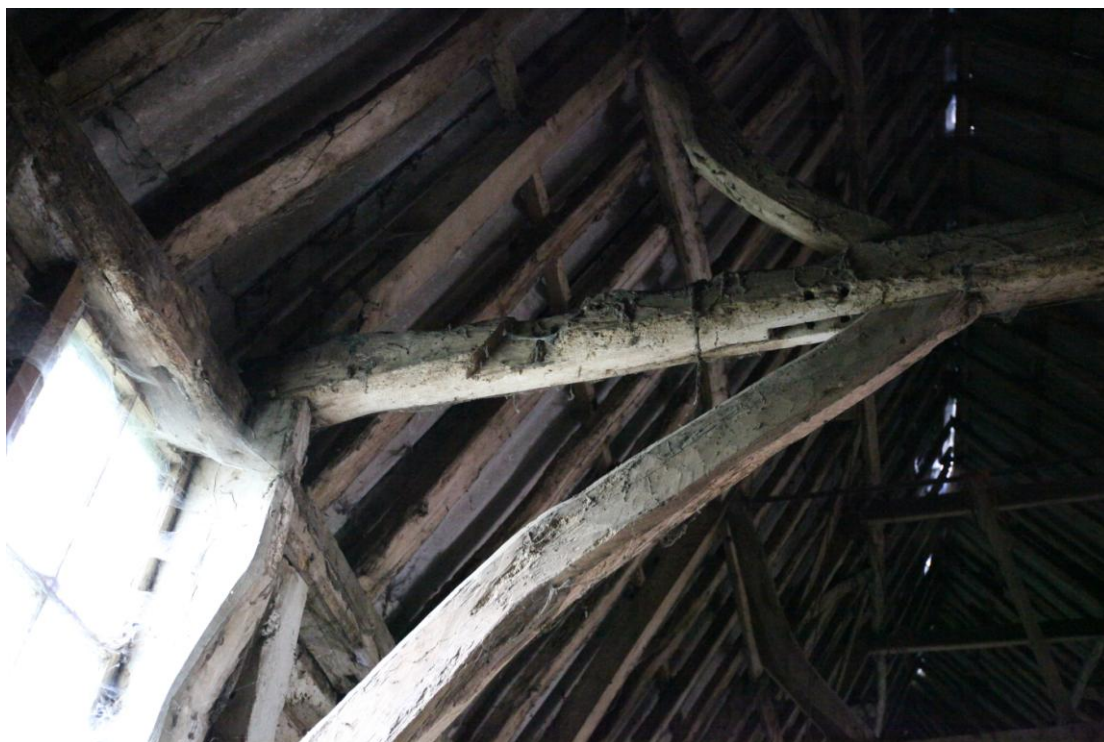
Illus. 10. The western end of the re-used tie-beam between bays G and F seen from the south, showing a trench for a passing brace of a type normally associated with barns of the early-14 th century or before. An identical trench occurs at the opposite end of the same timber (as would be expected), but while many studs and roof-plates show similar indications the majority of the remaining tie-beams appear to be primary.
