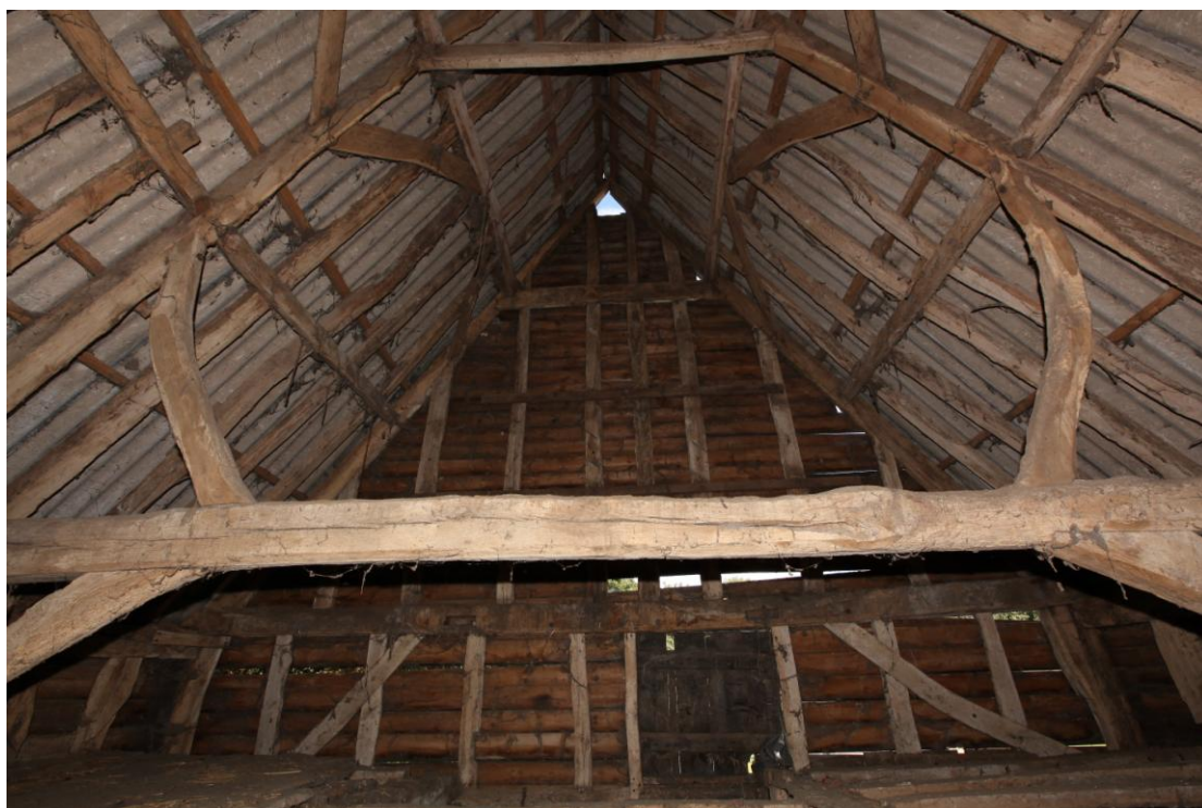
Illus. 9. The interior of the northern hay loft (bays A and B) from the south, showing the raking queen struts to the re-used tie-beam (with passing-brace trenches to left and right) and a loading hatch in the gable. The wind-braces extend to the gable in contrast to those of the main threshing barn.
