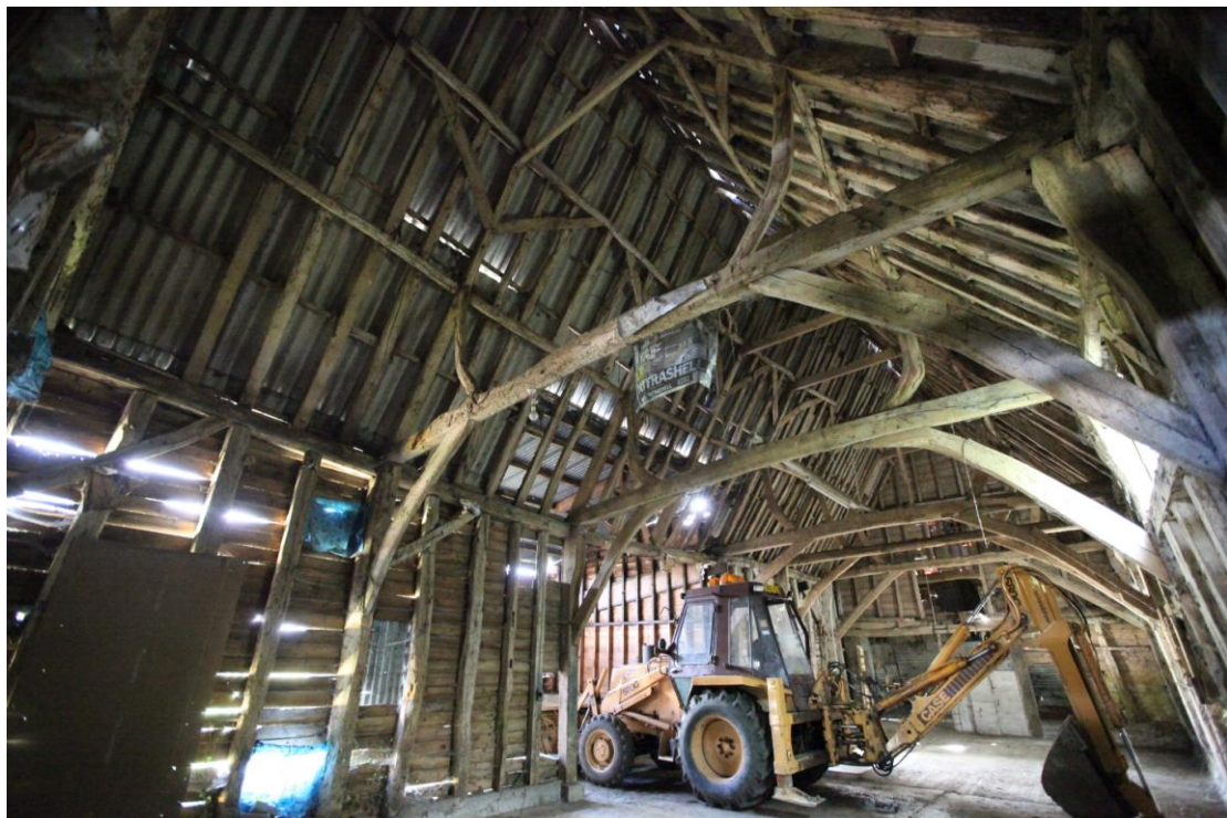
Illus. 4. A general view from the north-west of the main threshing barn (bays C-G) between the two stables, showing a tractor parked in the central threshing bay (E). The tie-beam between bays C and D in the foreground has trenches for passing-braces at both ends and has been re-used from an early-14 th century or earlier building.
