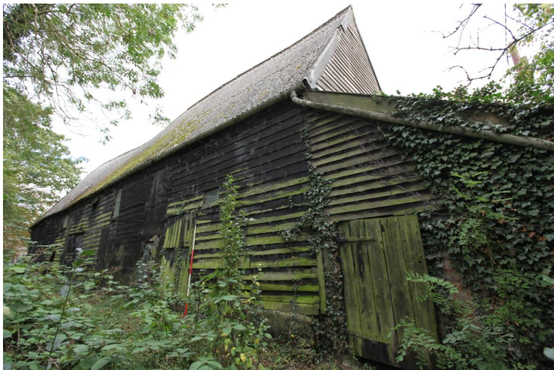
Illus. 2. The western exterior from the south-west showing the half-hung door to the southern stable (bays H and I) with the entrance to the 20 th century lean-to against the southern gable to the right.
