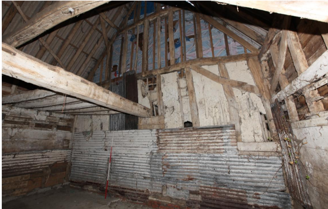
Illus. 11. The southern internal gable showing early wattle-and-daub and the remaining section of hay loft to the left. A hay rack and manger would have been attached to this gable, as indicated by a hay drop (narrow gap) in the ceiling of the loft immediately above.
