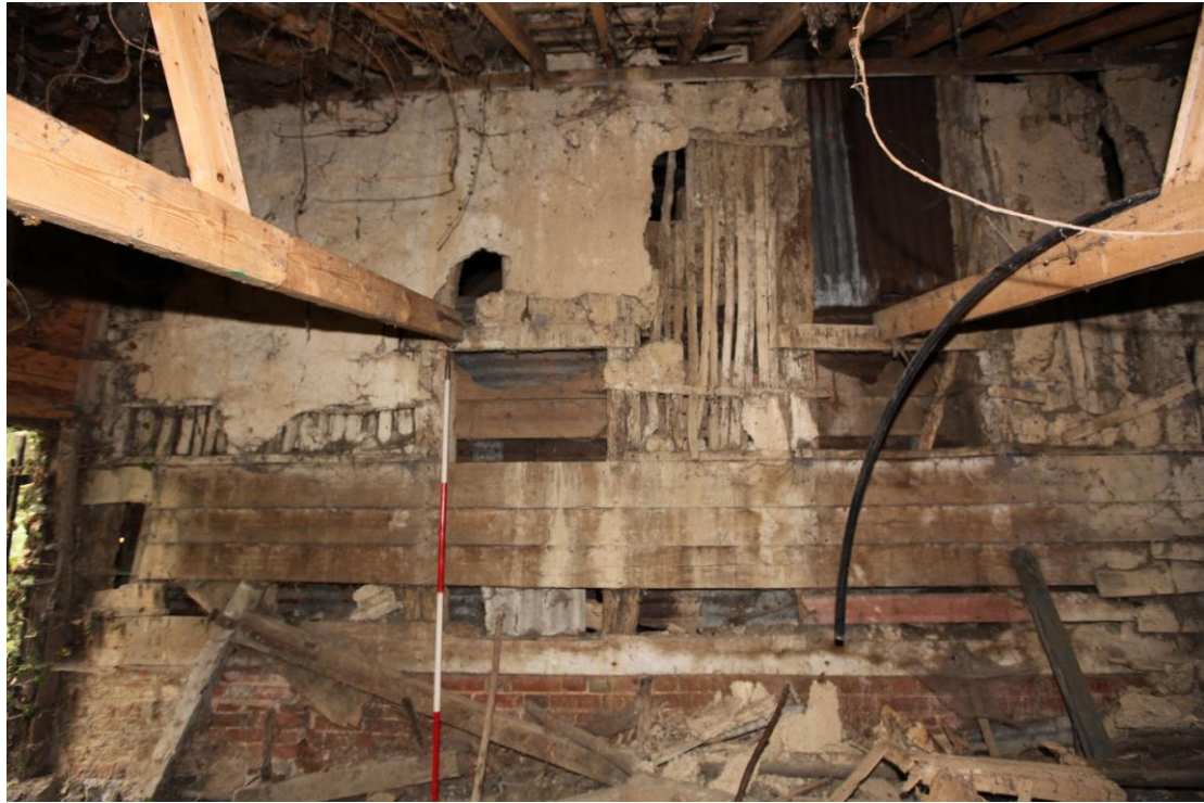
Illus. 3. The exterior of the southern gable preserved in the lean-to shed, showing the 18 th or early-19 th century ‘two-tier’ cladding of wattle and daub above weatherboarding. The entire barn is likely to have been clad in this manner before the addition of the present tarred weatherboarding.
